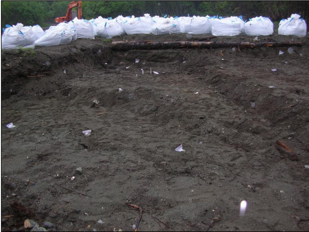
Photograph 5. Former Diesel AST Area showing screening samples and PCS filled Super Sacks®.
