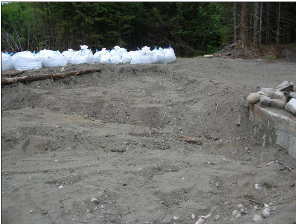
Photograph 4. Former Diesel AST Area excavation. Looking northeast.
