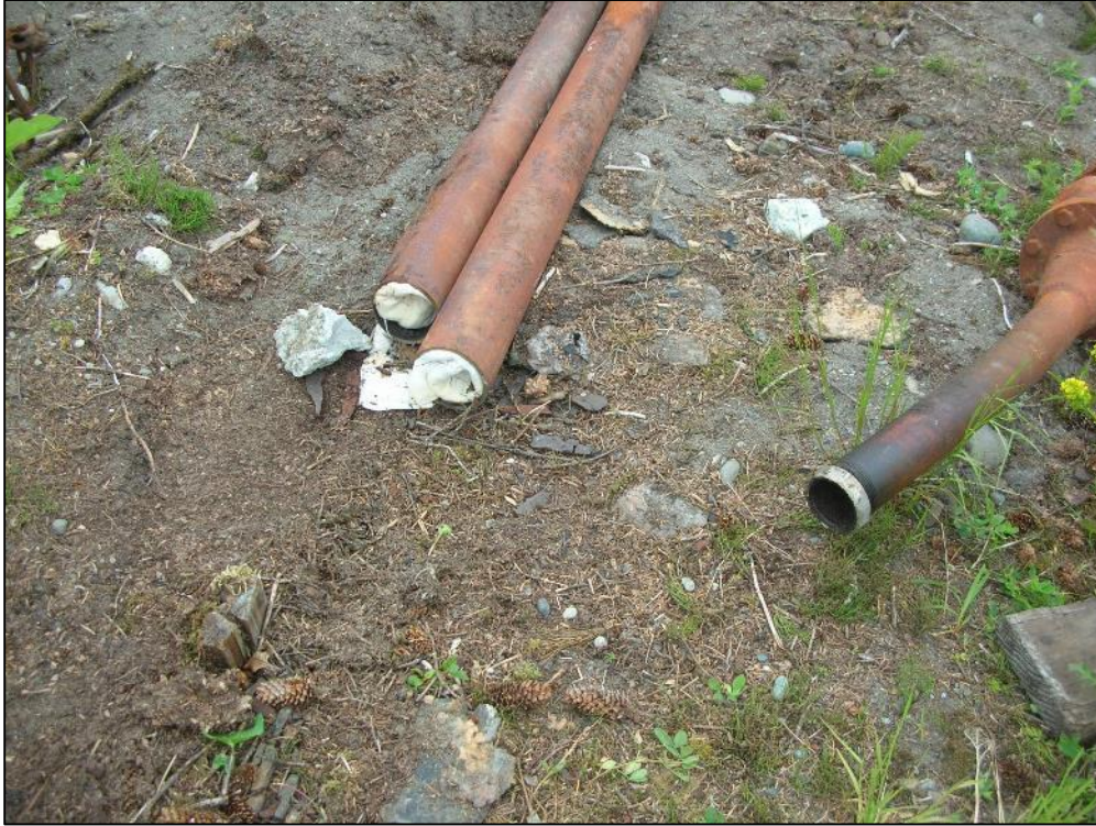
Photograph 9. Removed piping from the Former Fuel Pumphouse Area.
