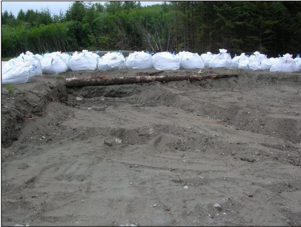
Photograph 3. Former Diesel AST Area excavation. Looking northwest.
