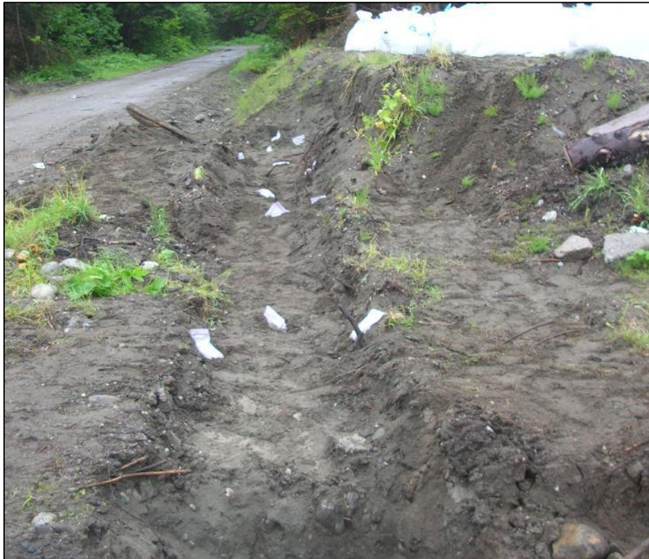
Photograph 8. Former Diesel AST Area showing screening samples in trench area.
