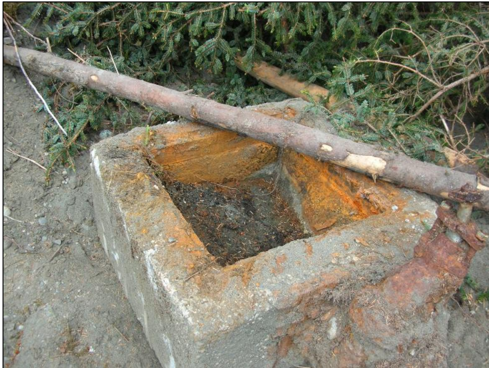
Photograph 6. Drain Area concrete catch basin after removal.
