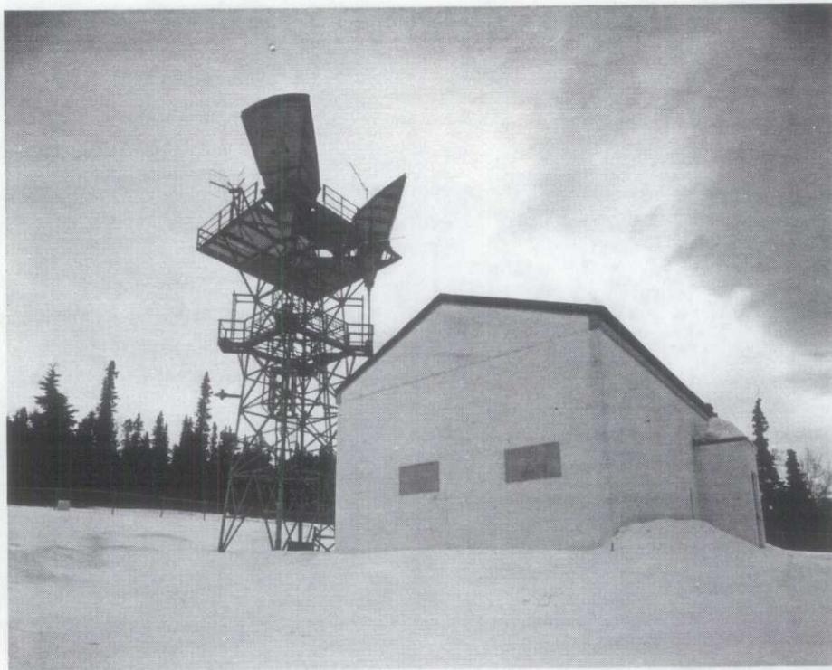
2. Radio relay building, view to southeast, showing TD-2 tower.
