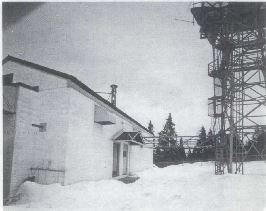
5. Entry of waveguides into building.
