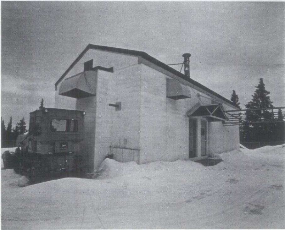
1. Radio relay building, view to northwest.
