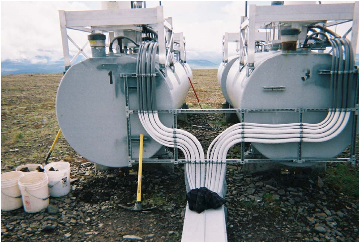
Excavation beneath AST 1 valve completed looking south.
