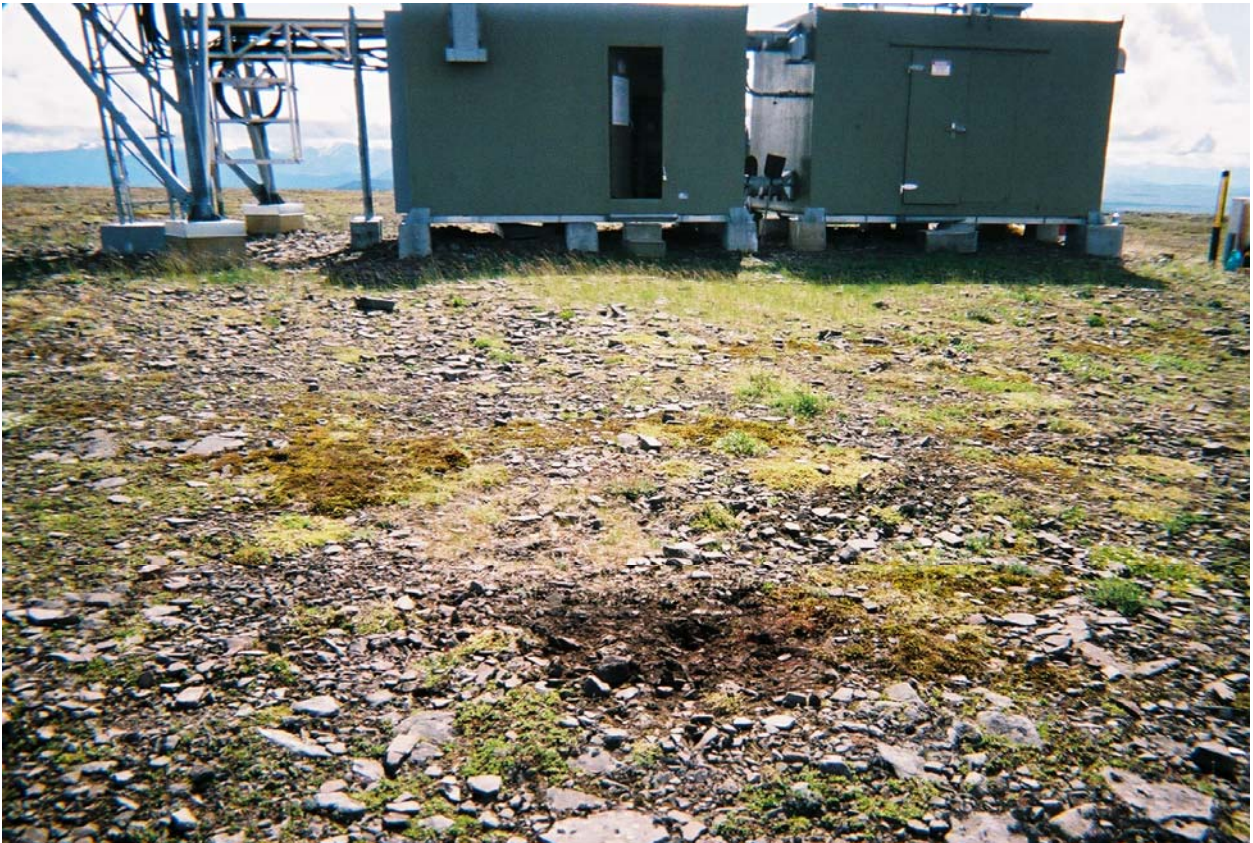
Completed excavation and backfill of Burn Pit 1 looking south.
