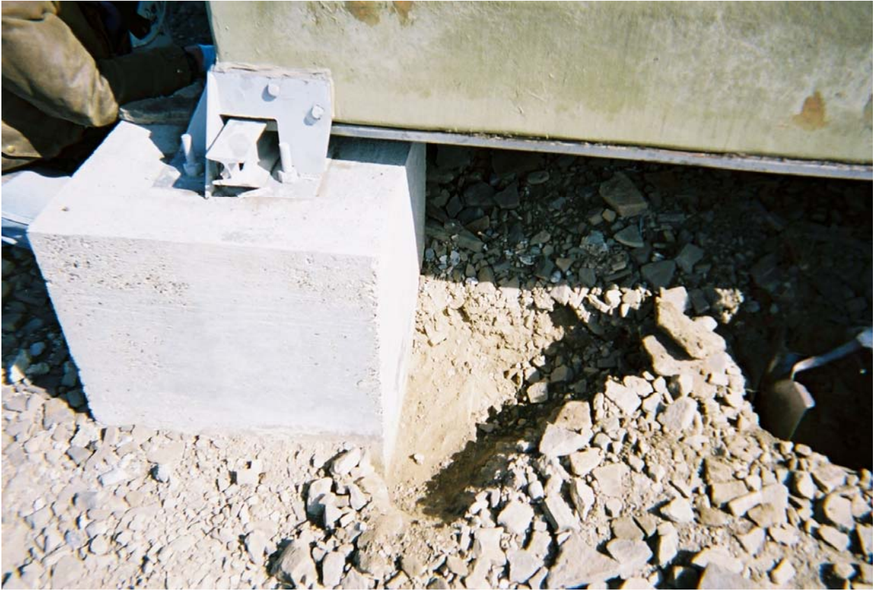
Excavation beginning beneath northwest corner of the Generator Module.
