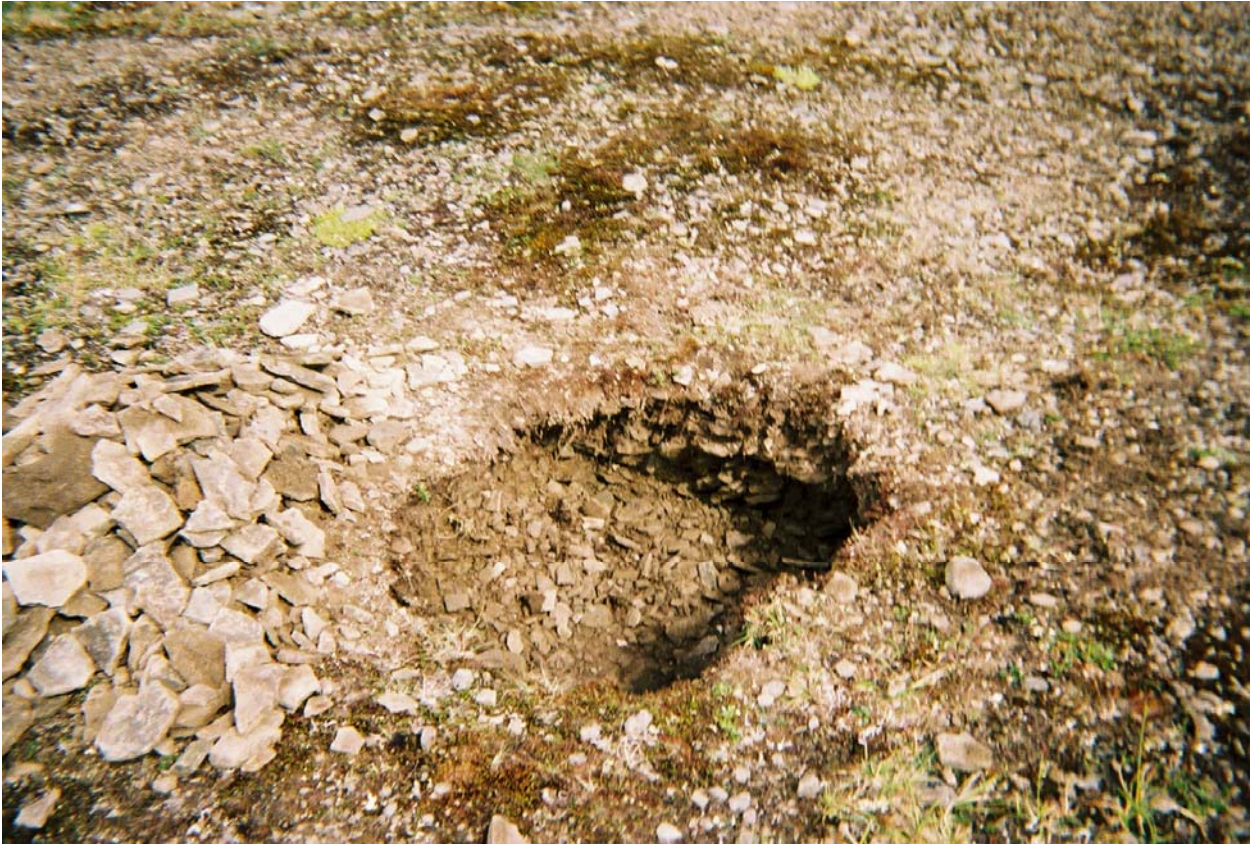
Final excavation of fuel bladder staging area looking north.
