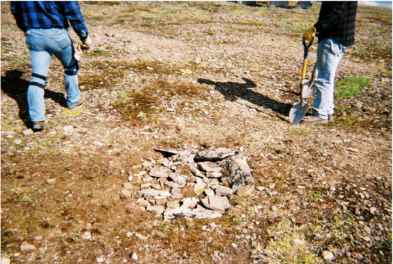
Fuel bladder staging area excavation backfilled with native material looking northeast.
