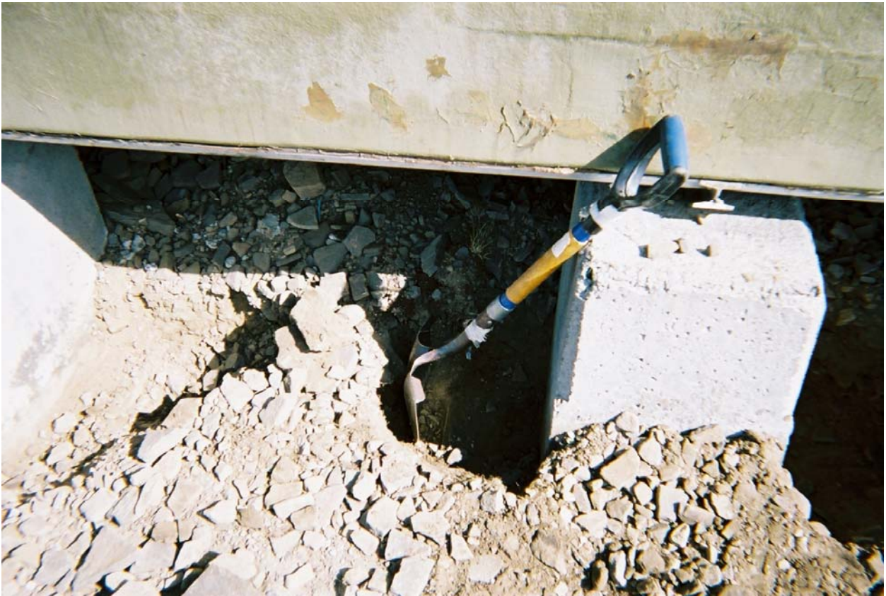
Excavation continuing along western edge of the Generator Module.
