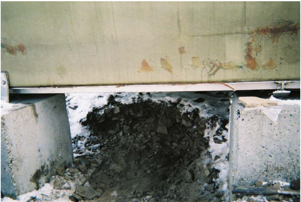
Completed excavation beneath northwest corner of the Generator Module. Slope
