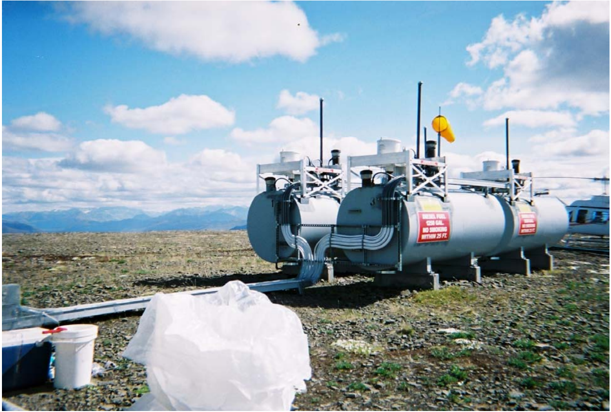
Site photograph of Slope Repeater AST area; view looking southeast.
