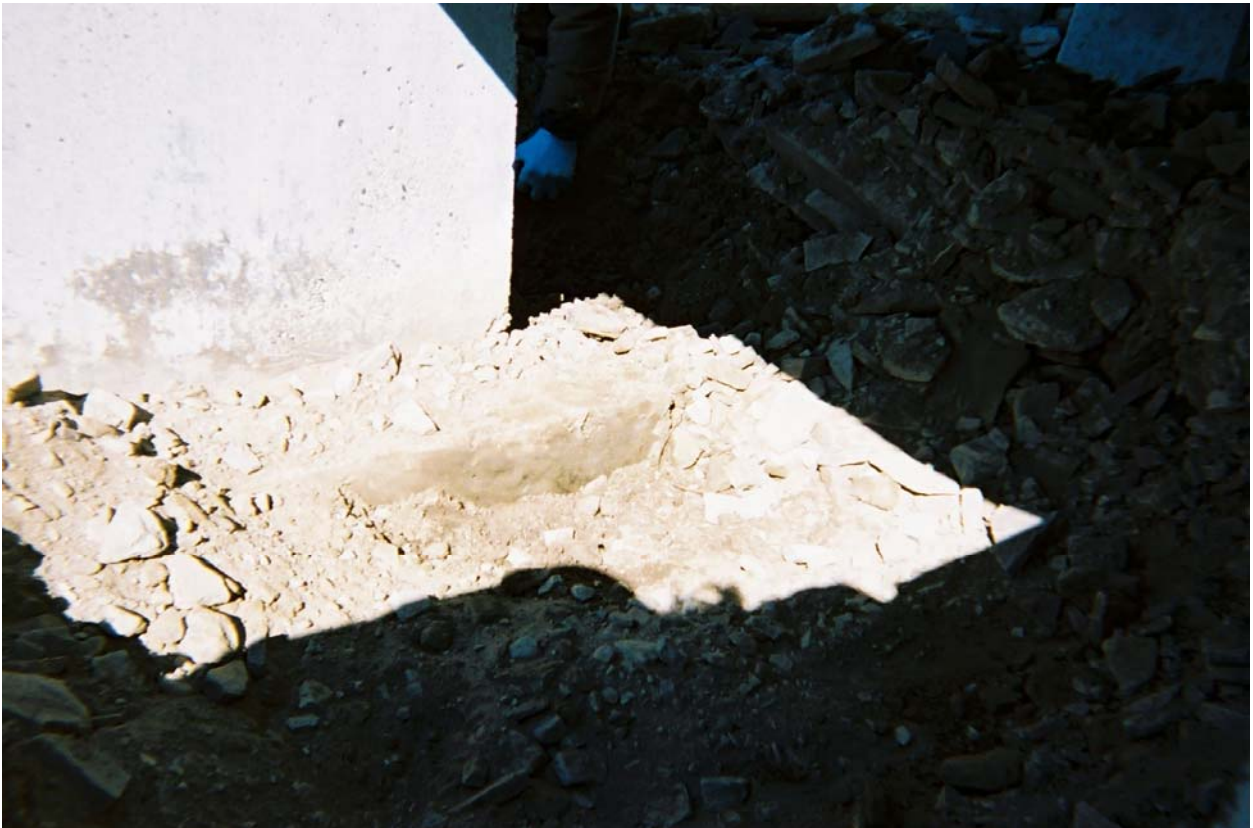
Completed excavation beneath northwest corner of the Generator Module.
