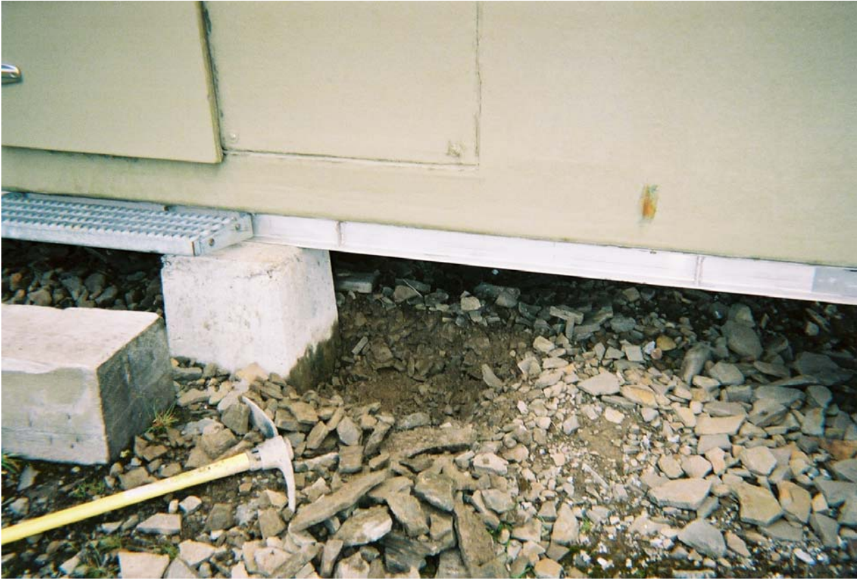
Excavation beneath north side of the Generator Module looking south.
