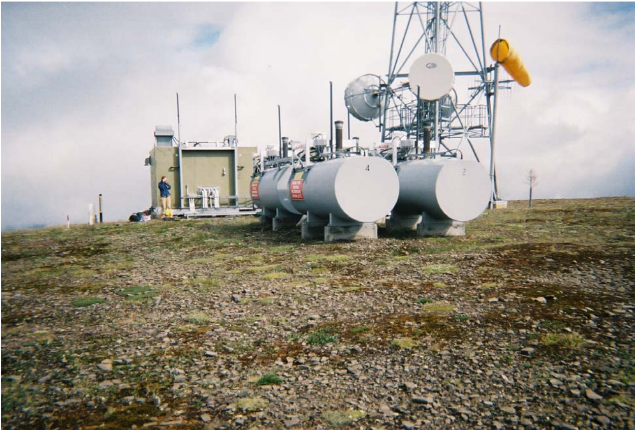
Site photograph of Slope Repeater AST area; view looking northeast.
