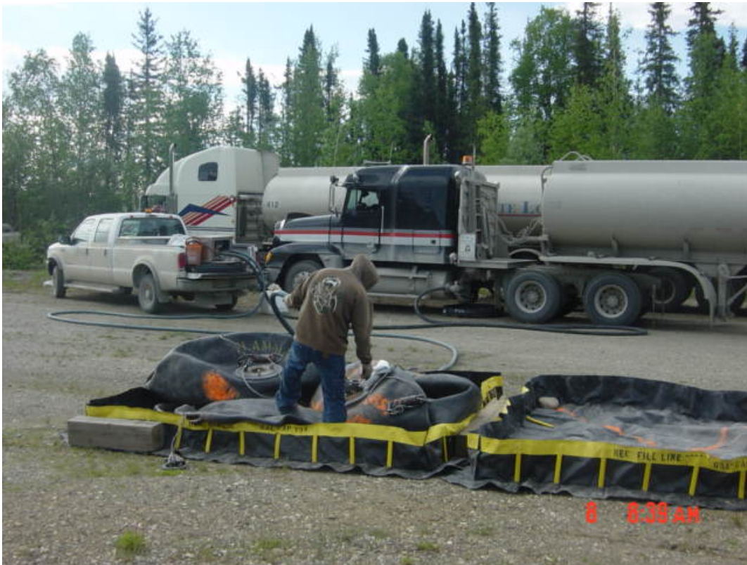
Highway site staging area. Filling fuel bladders within portable secondary containment
