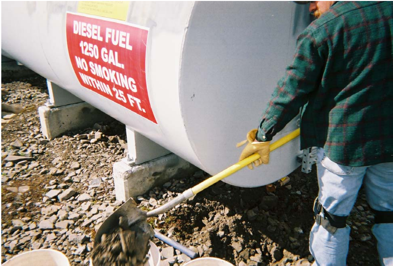
Excavation beneath AST 1 valve in progress looking southwest.
