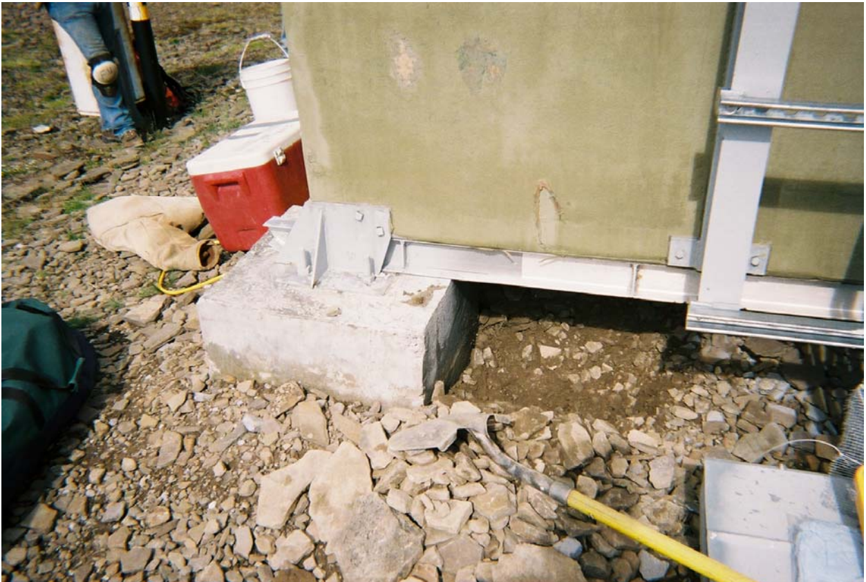
Excavation in the southwest corner of the Generator Module looking north.
