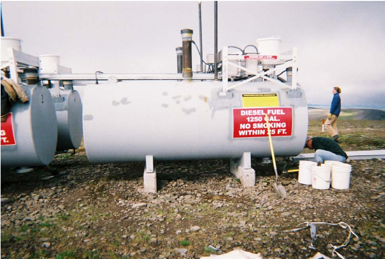
Excavation in progress beneath AST 1 valve looking west.
