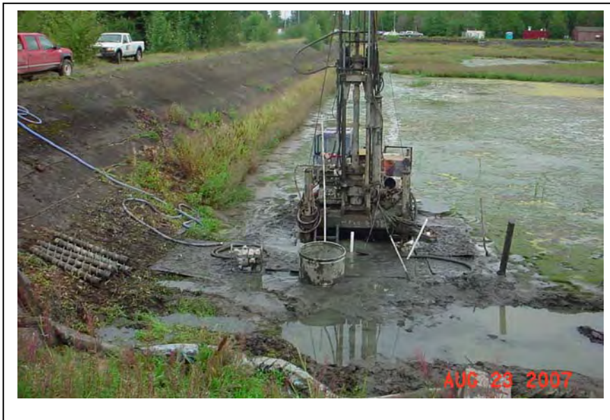
Photo 2: A view of the drill rig while installing Temporary Well TW1; looking east (August 23, 2007).
