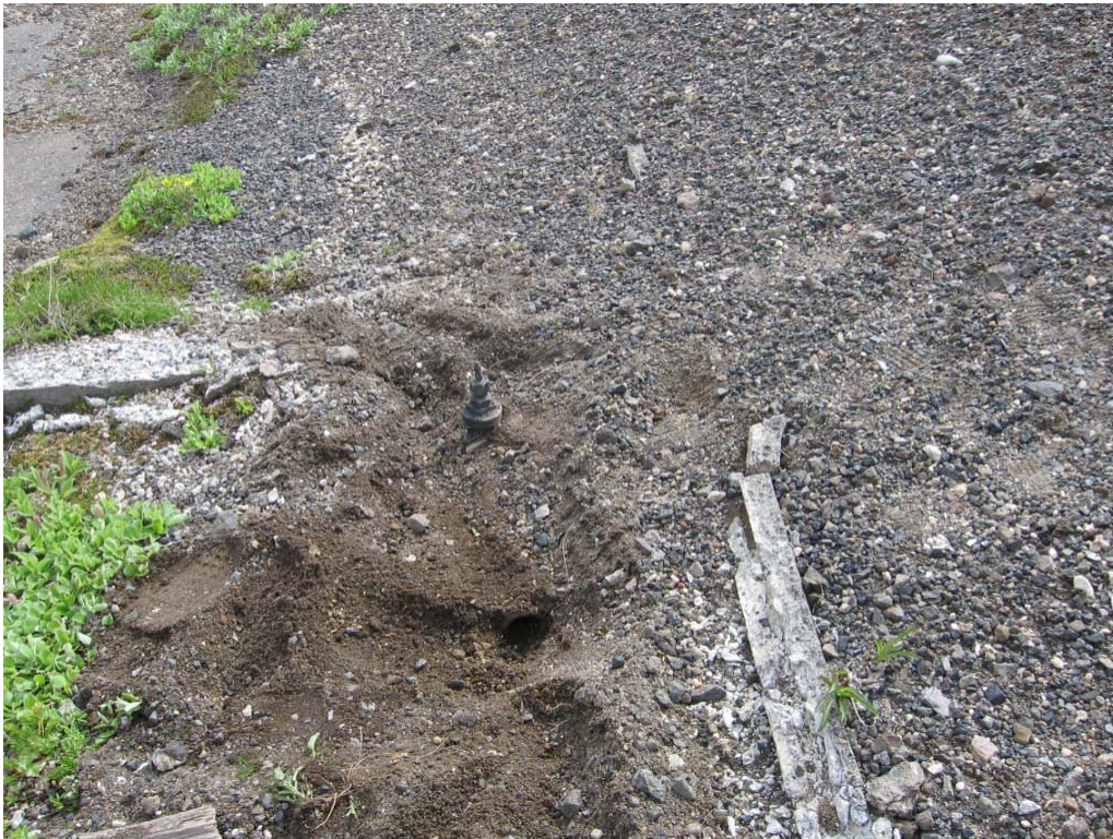
Looking at concrete foundation at infirmary area. (23 June 2010)
