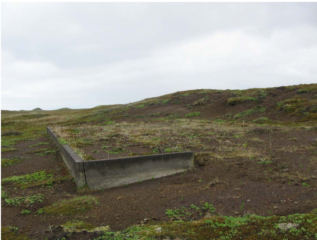
Looking north at warehouse foundation with concrete footings. (23 June 2010)
