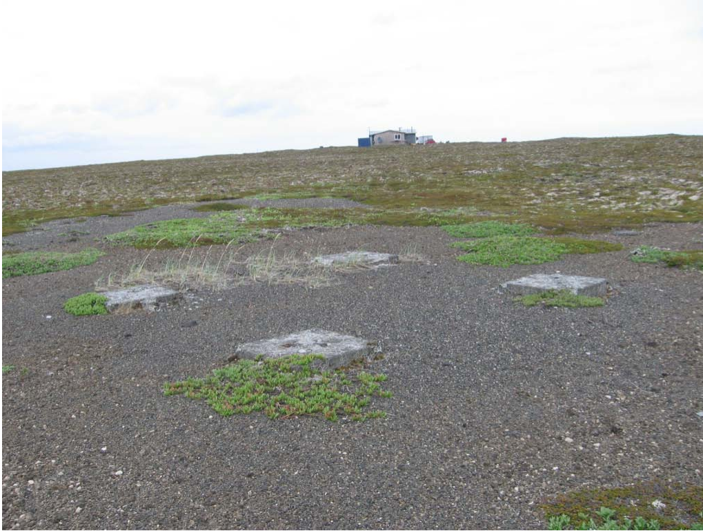
Looking northwest at C.A.A. Range Station antennae foundations. (24 June 2010)
