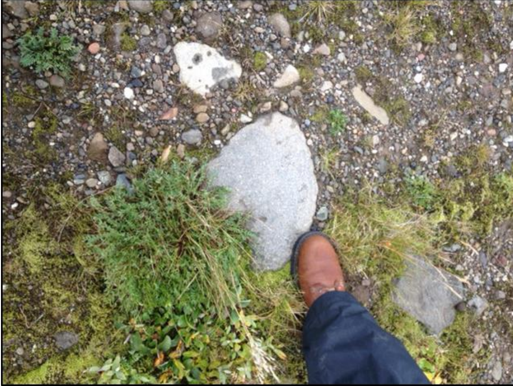
Figure 5-1. Impenetrable Soil at Feature M-RD-001.
