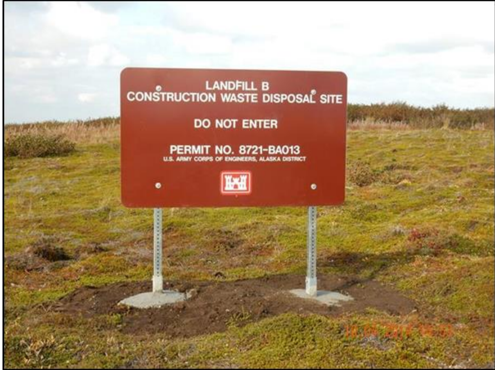
Figure 4-6. Installation of Signs for Landfill B Disposal Site.
