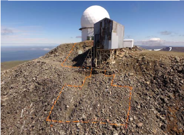
Figure 1-2. Site SS016 Upper Tram Terminal in front. Area to be excavated is marked in orange.
