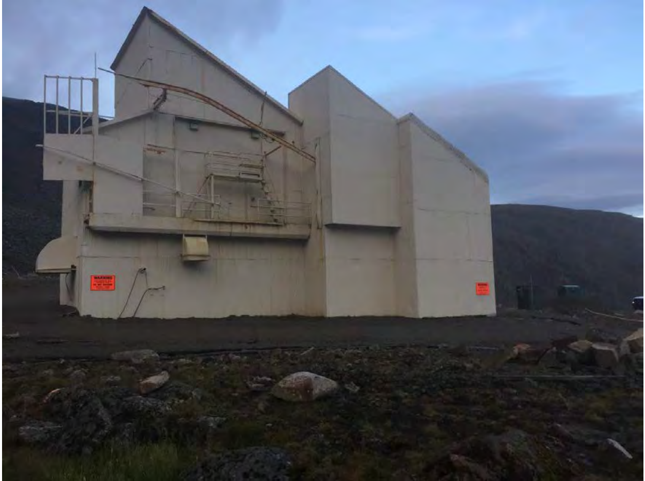
SS017 view south. LUC signage shown mounted to the lower tram building.
