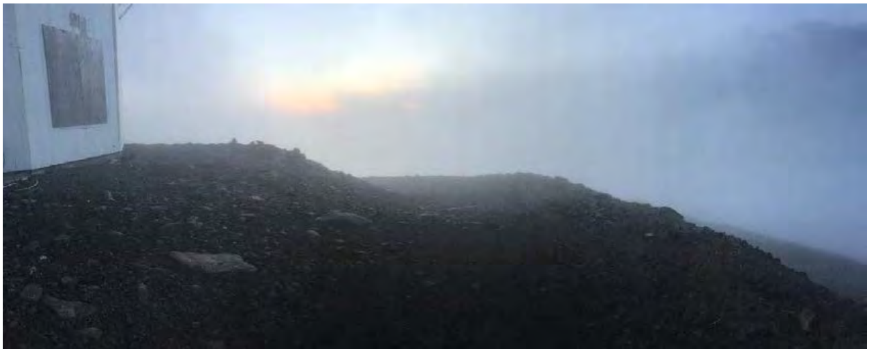
SS016 view north east below radome.
