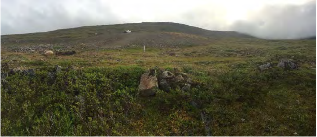
LF003 view north. CMW4 shown in foreground at toe of the landfill.
