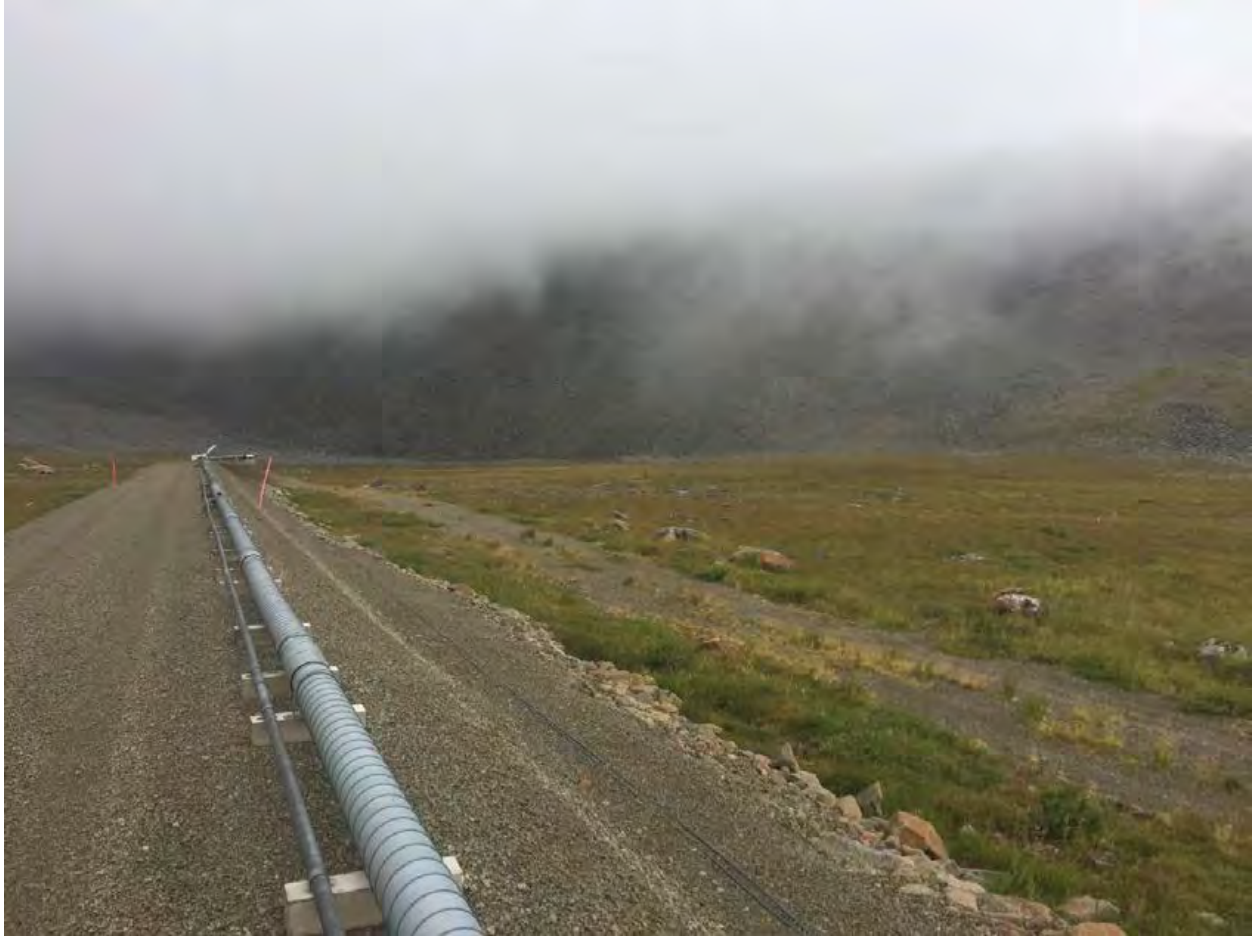
SS013 view north east. Site overview.
