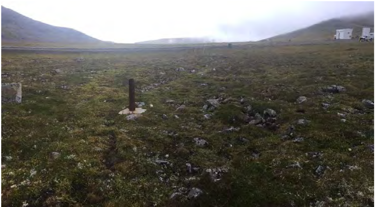
Site SS015 view south west. WW6 shown in foreground. Water transmission line pad and pump building shown in background.
