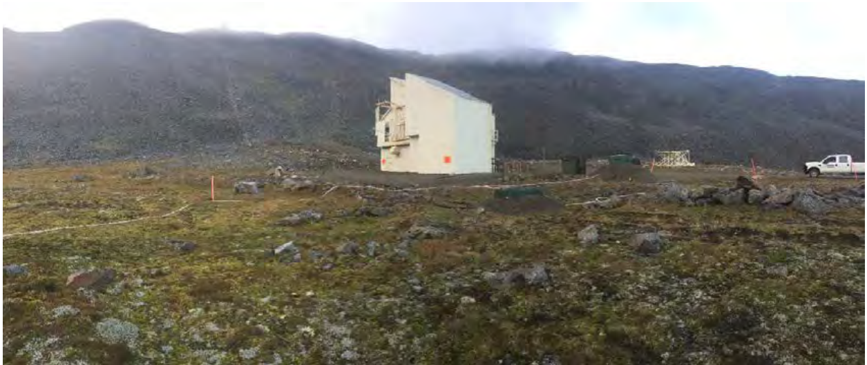
SS017 view east. Lower tram building and LUC signage shown.
