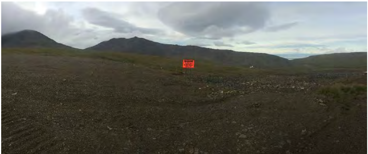
LF003 view south. Western LUC signage and landfill cap shown.
