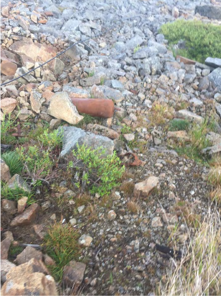
LF003 view east. Debris daylighting along western toe of the landfill.
