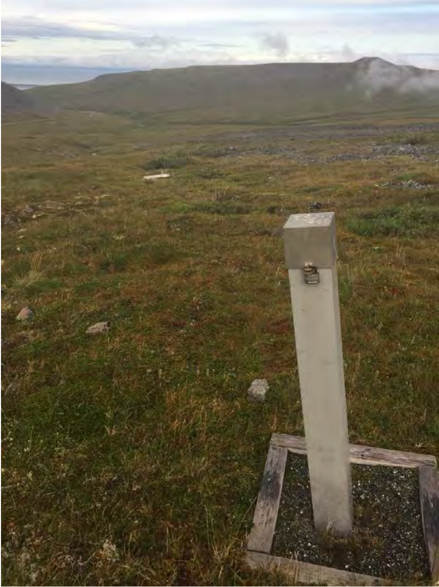
LF003 view west. Close-up of CMW6.
