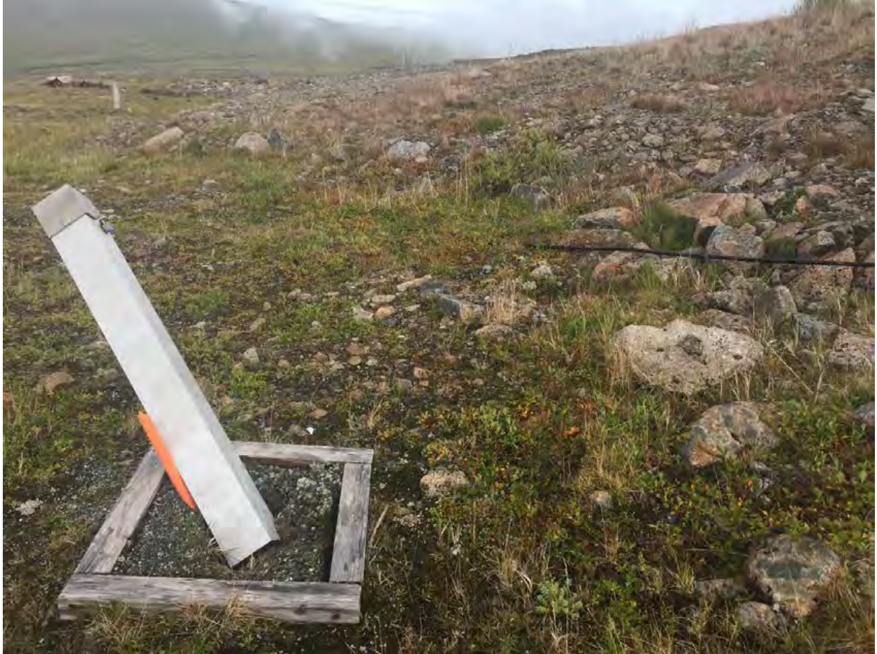
LF003 view west. CMW3 shown in foreground along toe of the landfill at photographs right.
