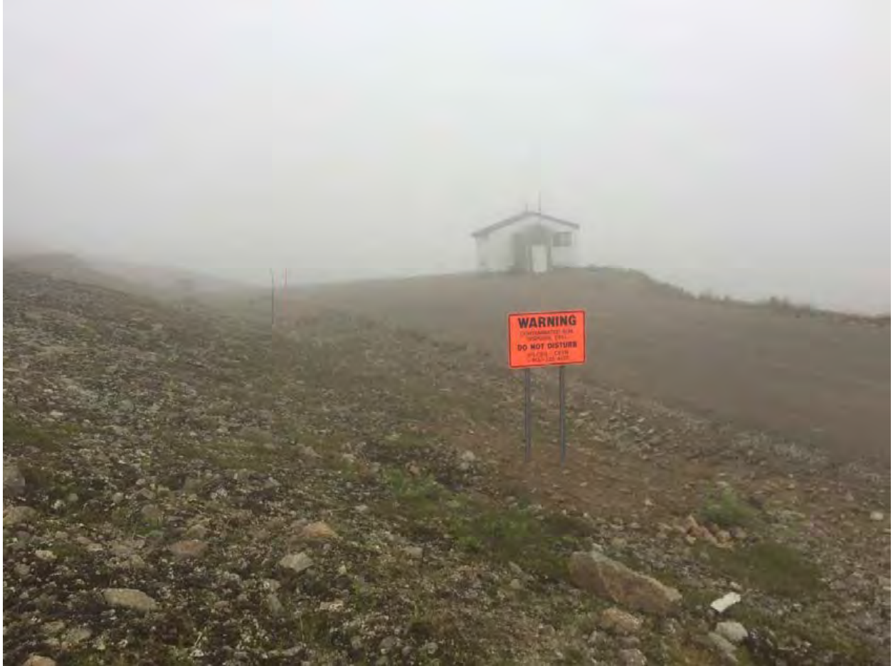
SS010 view south. LUC signage shown in foreground along site access road and Building 4104 shown in background.
