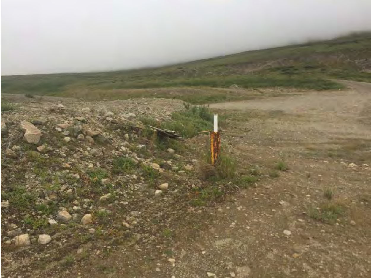
ST009 view north. MW5 shown in foreground. Also shown are the former borrow pit and biocell foundation.
