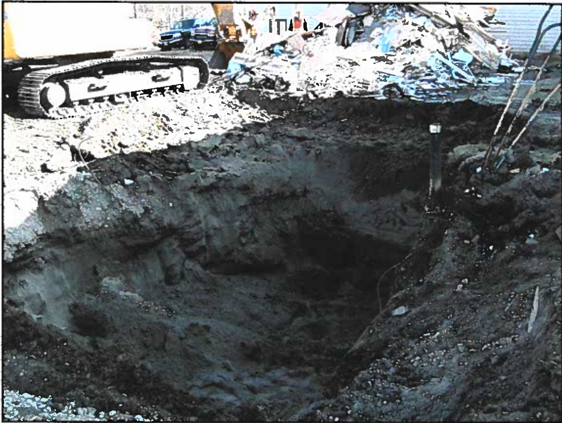
Photograph 7 Excavation Pit for 300-gallon UST
