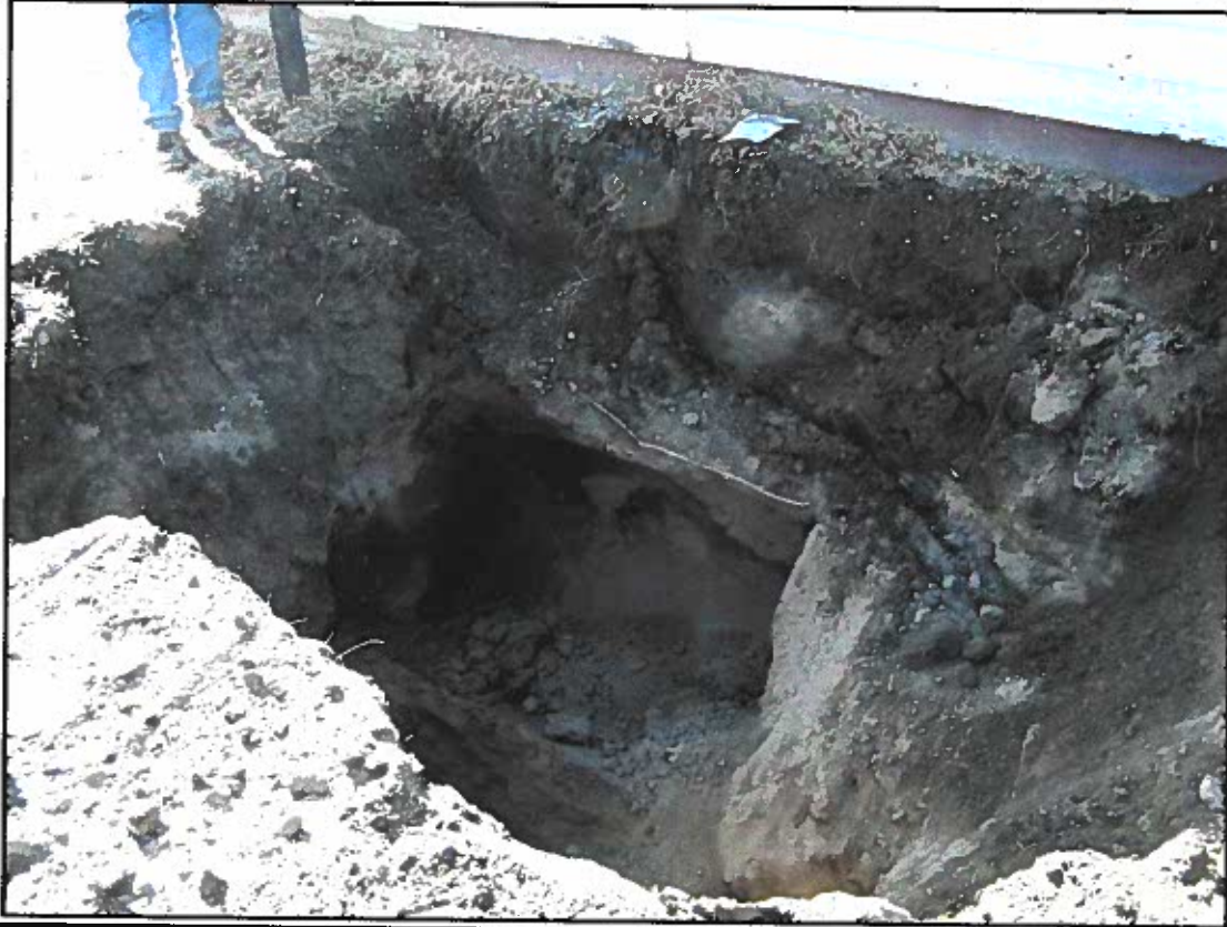
Photograph 3 Excavation pit for 1,000 gallon UST
