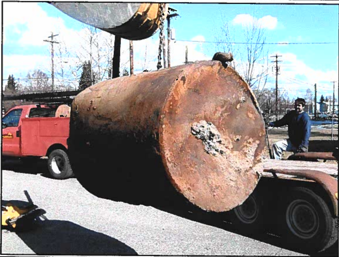
Photograph 5 Removed 1,000-gallon UST
