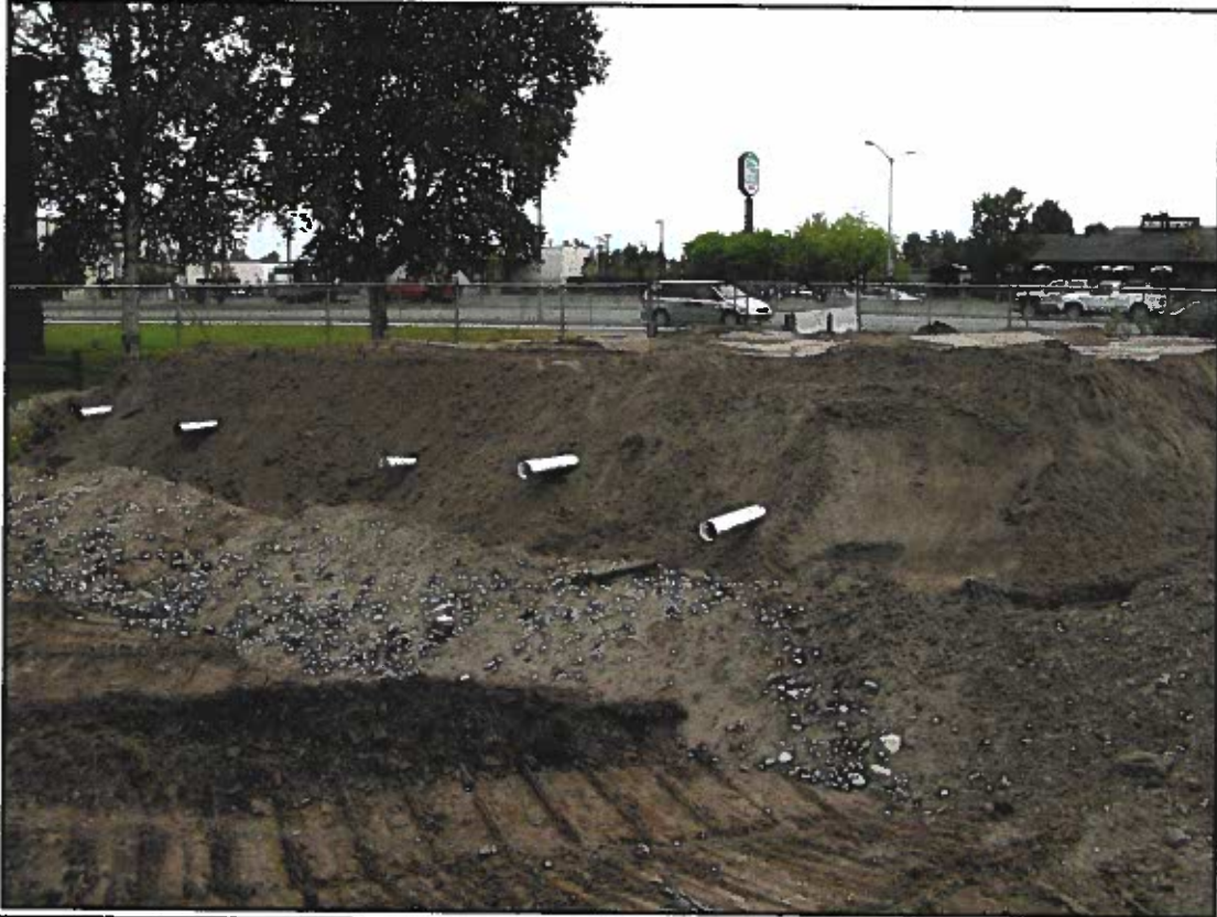
Photograph 11 Final excavation pit for 300-gallon UST
