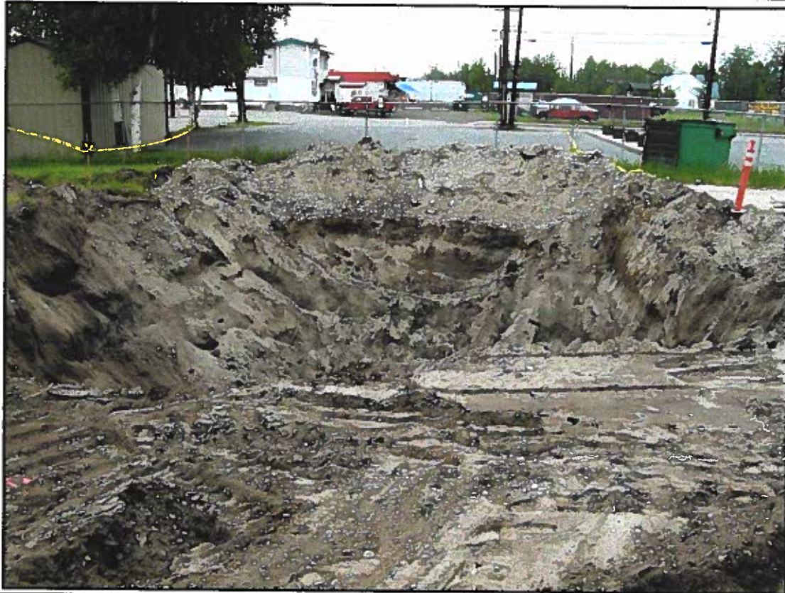
Photograph 9 Final excavation pit for 300-gallon UST
