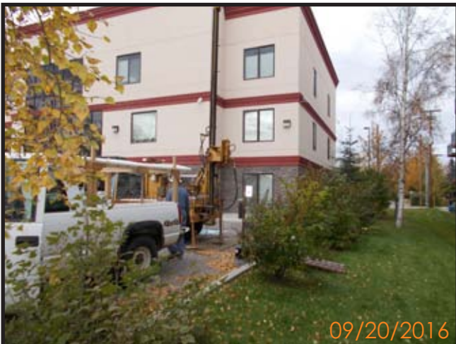
Photograph 5: Viewed North- The Drilling Company drilling/installing Monitoring Well, MW-1.
