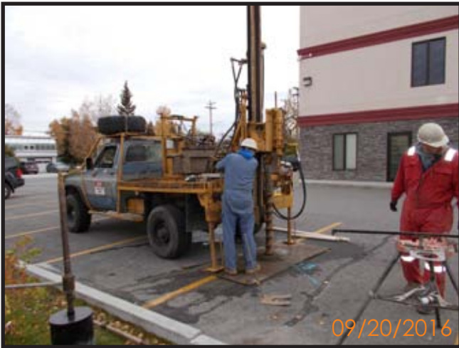
Photograph 1: Viewed Northeast- The Drilling Company drilling/installing Monitoring Well, MW-3.
