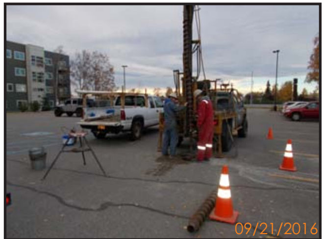
Photograph 10: Viewed South-The Drilling Company drilling/installing Monitoring Well, MW-2.
