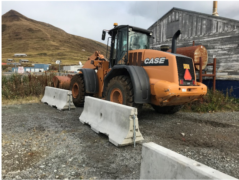
Loader scraping for MW-3, North-East
