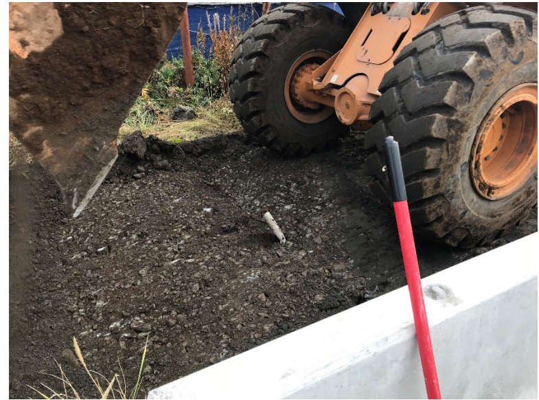
MW-3 exposed, East
