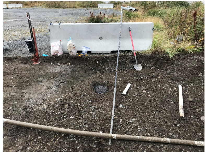
Decommission of MW-3 Complete, West
