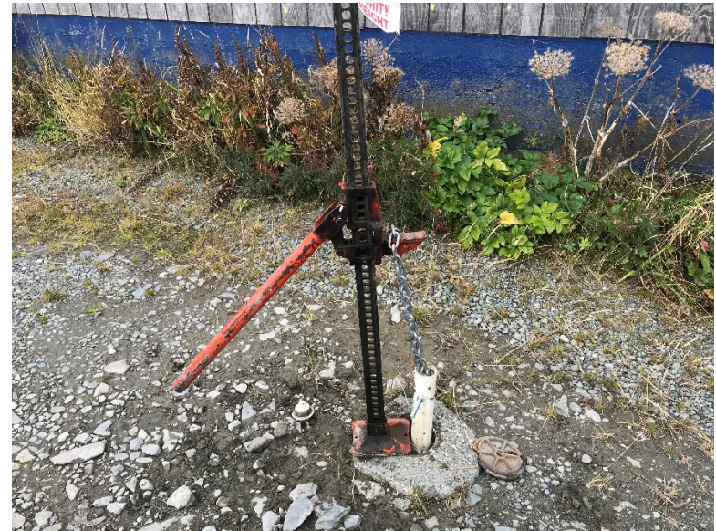
Removing MW-1, North-West
