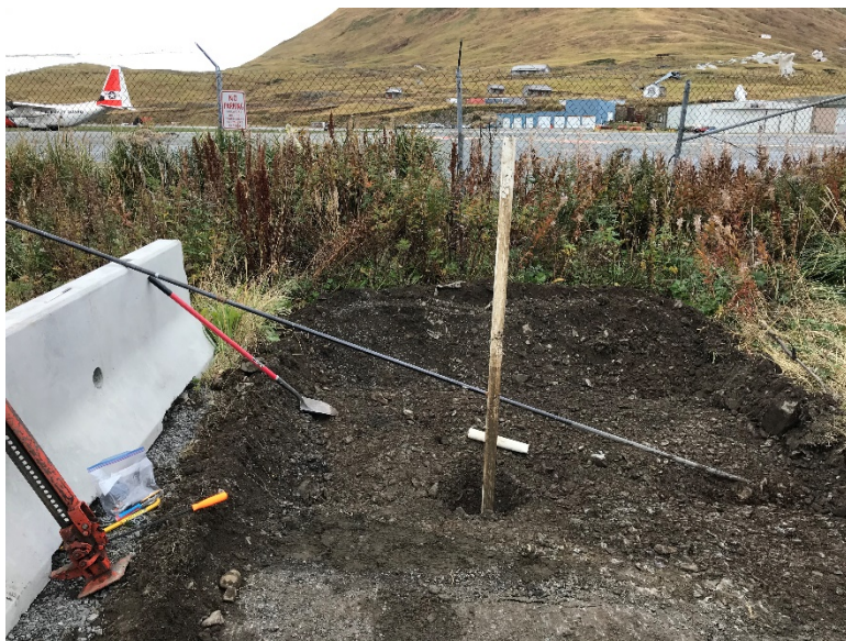
Removal of MW-3, North
