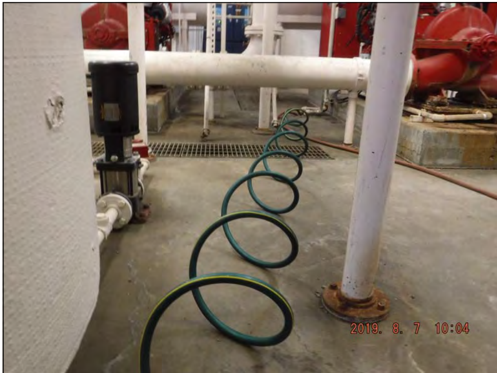
OU2 DRMO — Hose for purge water in the Building 5009 Well House (view N/A)
