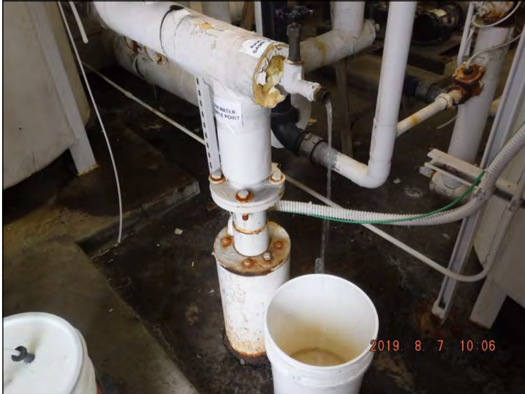
OU2 DRMO — Purge water prior to sampling of the WSW (view N/A)
