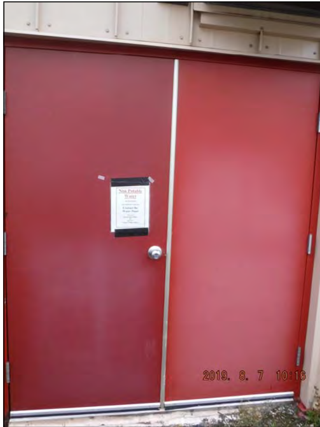
OU2 DRMO — Door at the Building 5009 Well House (view N)
