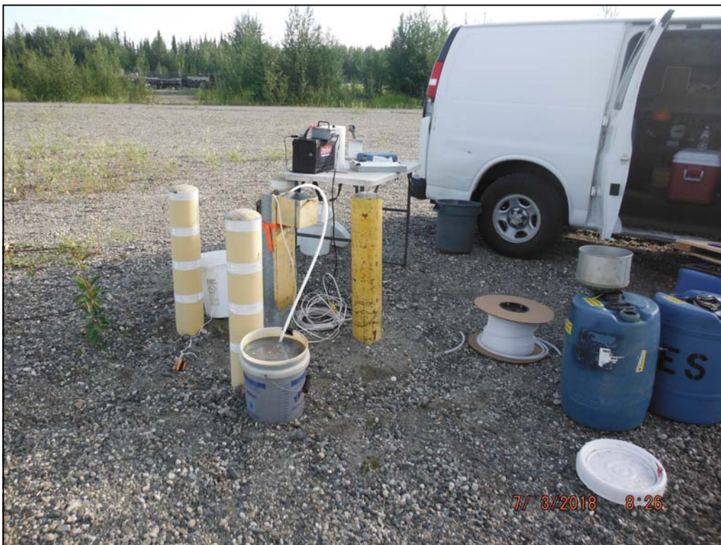
OU2 DRMO4 (3-Party) — Monitoring Well Development at AP-10445MW (view N)
