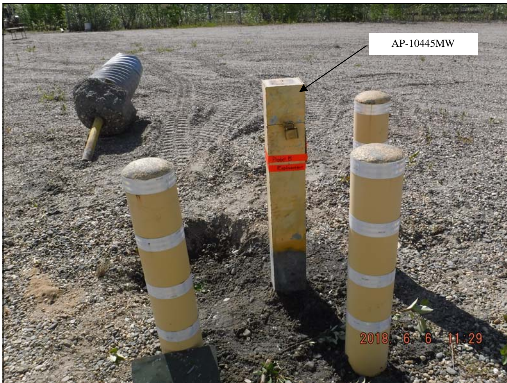
OU2 DRMO4 (3-Party) — Replacement Monitoring Well AP-10445MW (view S)
