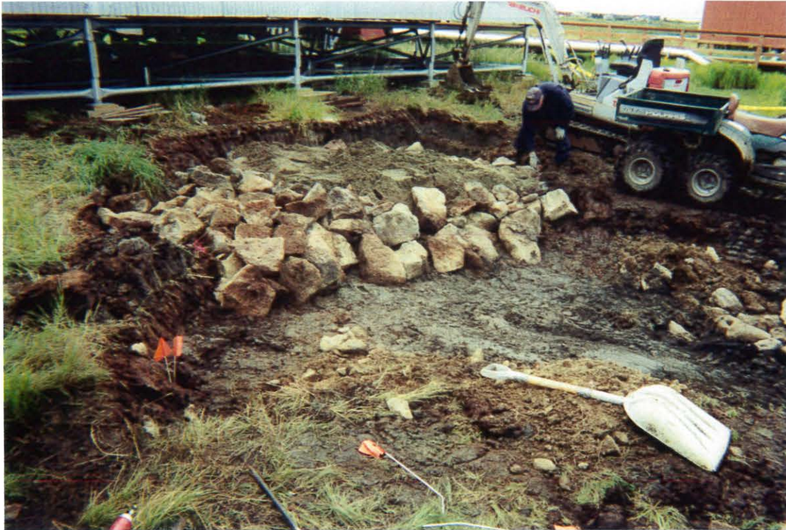
Area C excavation backfill activities. Photograph taken by Denise Daggett.
