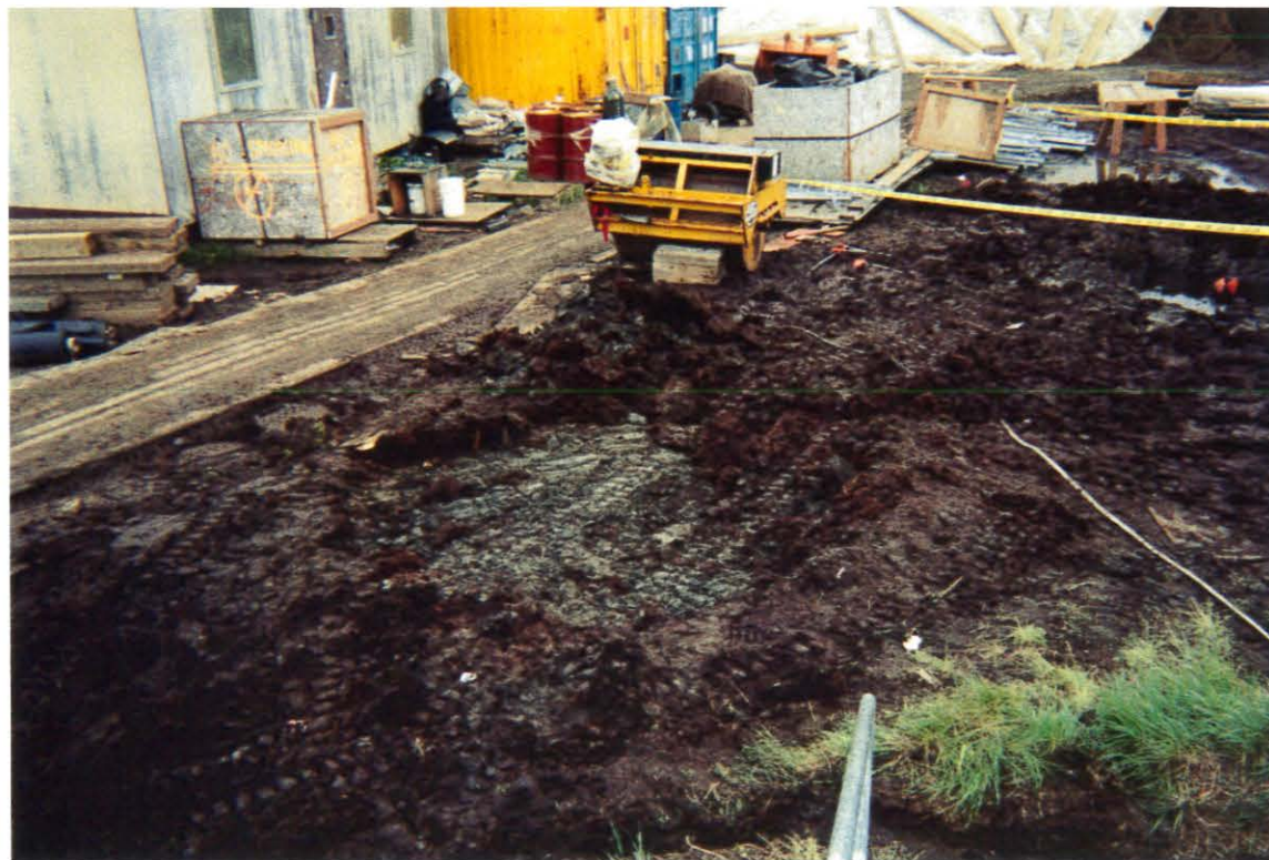
Area B excavation (middle of photo) and Area A excavation (right side of photo) following the removal of DRO contaminated soil. Photograph taken by Denise Daggett.
