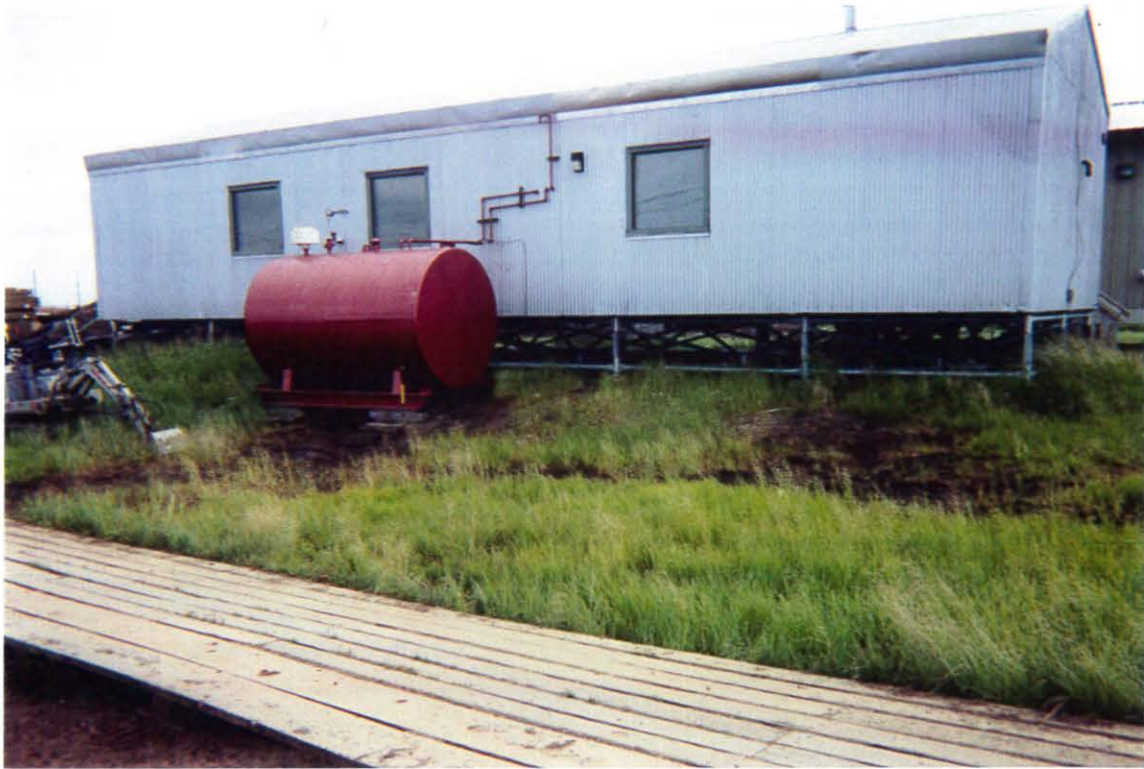
Area C and Area D excavations prior to the removal of DRO contaminated soil. Photograph taken by Denise Daggett.
