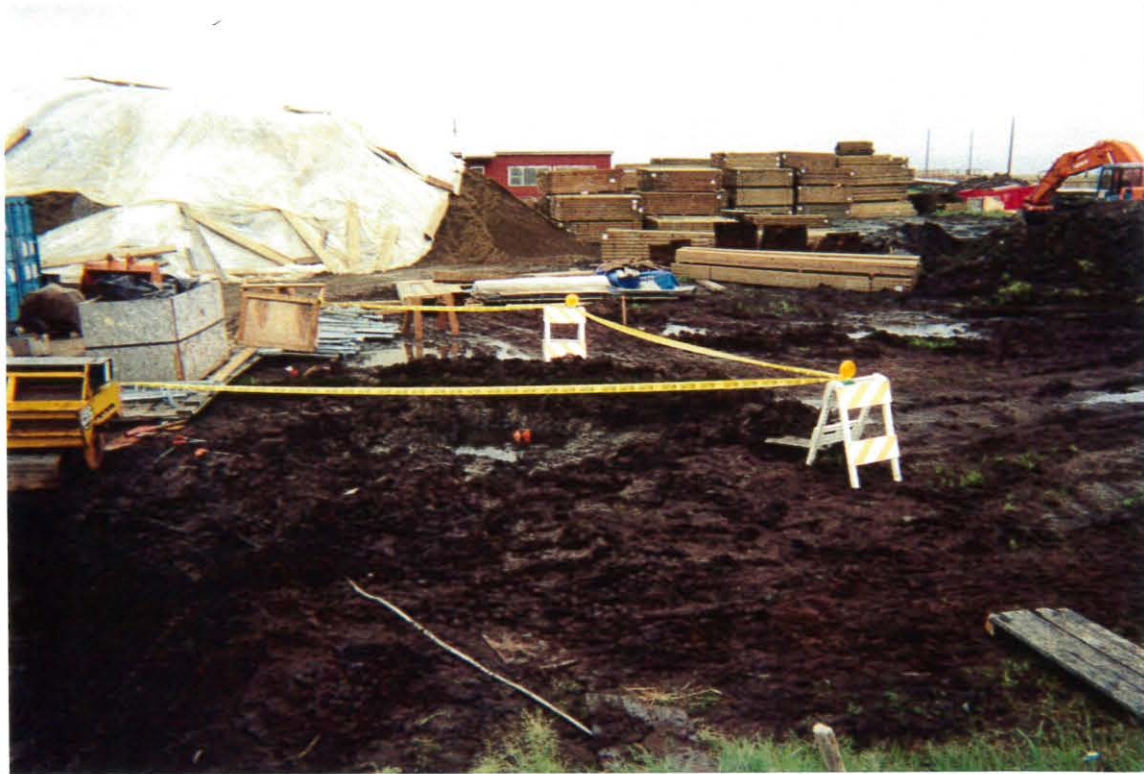
Area A excavation following removal of DRO contaminated soil. Photograph taken by Denise Daggett.
