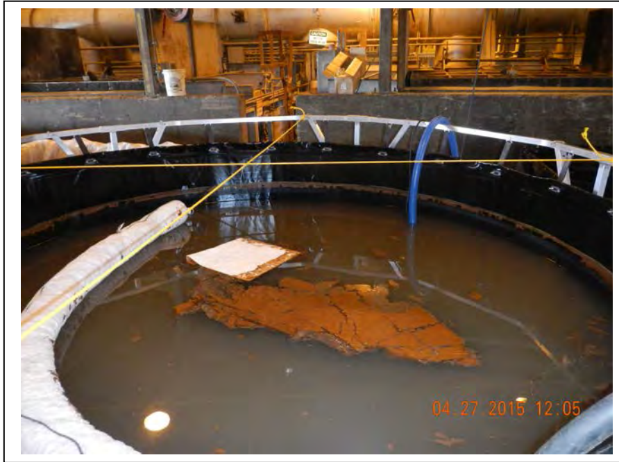
Photo 17: Pre-treated sump water in the round 1,600-gallon holding tank. (April 27, 2015).
