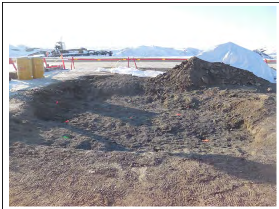
Photo 12: We collected analytical soil samples from the base and sidewalls of the excavated area; facing northwest towards Stevenson Street. (April 18, 2015)
