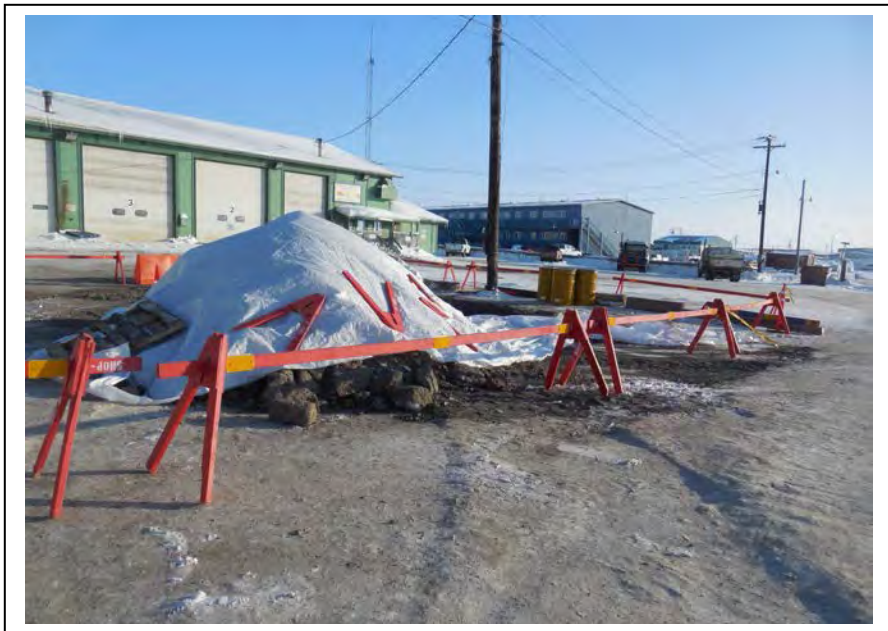
Photo 10: Excavated soils were stockpiled in the northeast corner of the fuel release area (E1). We collected five field-screening samples from the soil stockpile; facing south. (April 17, 2015)
