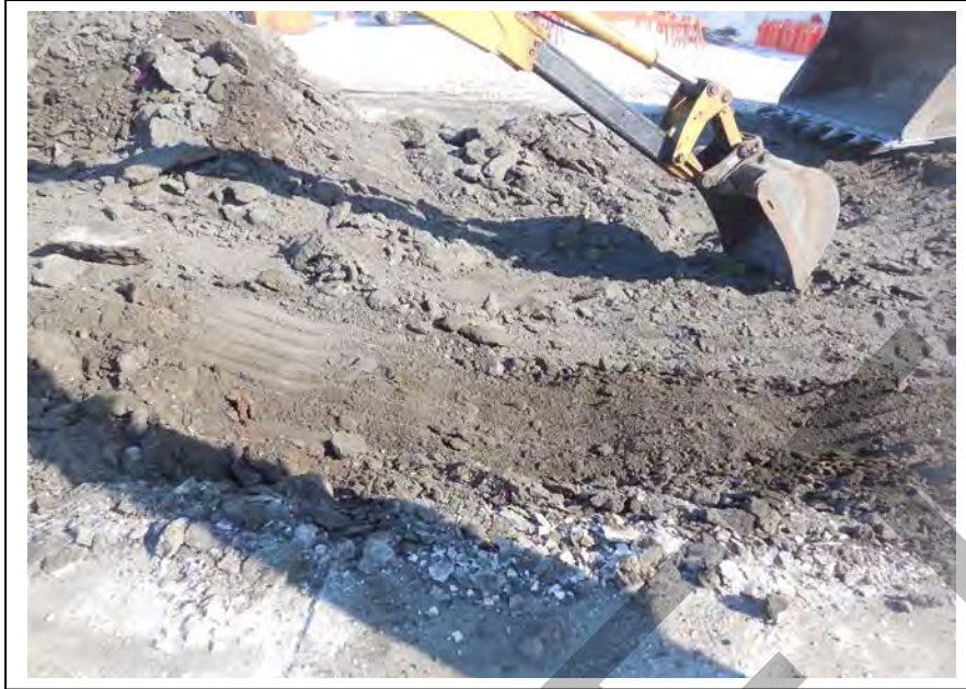
Photo 11: Staining was observed in the west corner of the fuel release area (E1); facing east (April 17, 2015).
