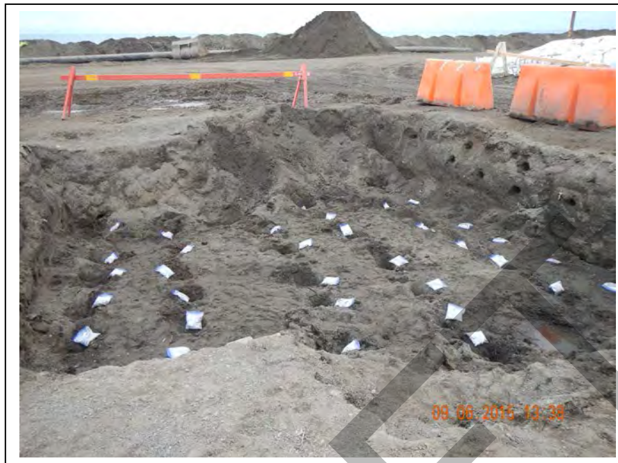
Photo 40: Field screening the base of excavation and NE sidewall; facing north (September 6, 2015).
