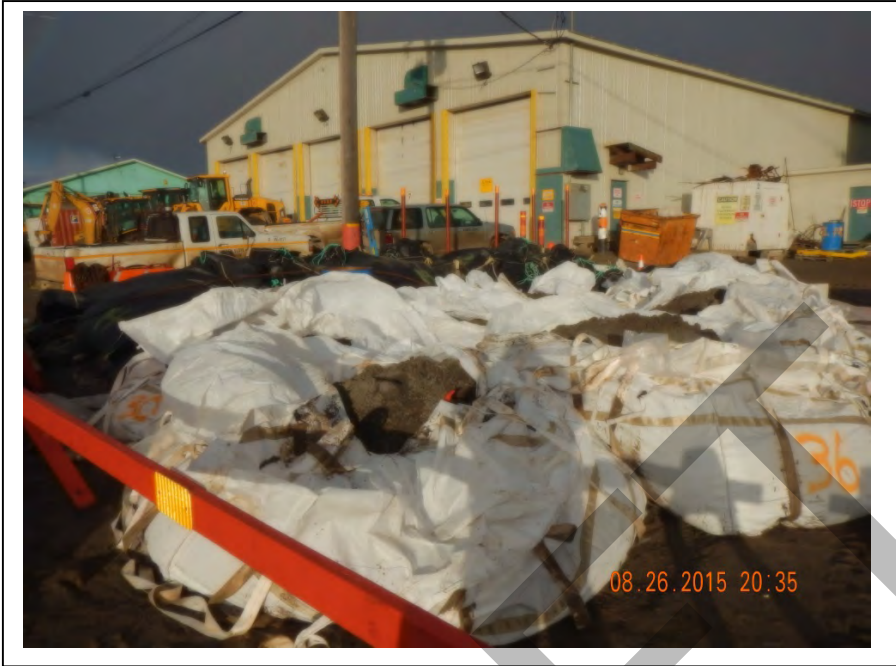
Photo 32: Supersacks containing potentially-contaminated soil removed from the excavation site (August 26, 2015).
