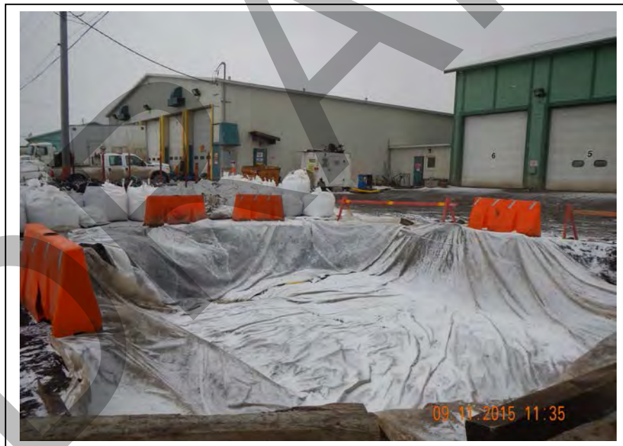
Photo 45: Site covered to prevent fresh snow from contacting exposed soil; facing east (September 11, 2015).
