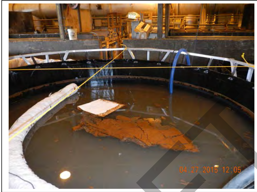
Photo 17: Potentially-contaminated sump water contained in a 1,600-gallon FASTANK (April 27, 2015).
