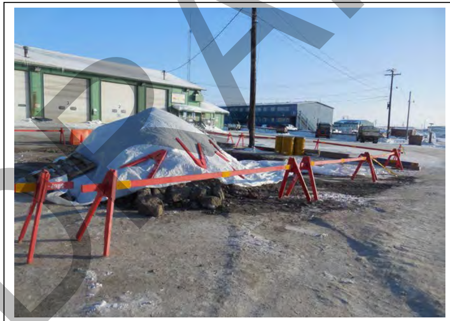
Photo 10: Excavated soil was stockpiled in the northeast corner of the fuel release area (E1). Five field-screening samples were collected from the soil stockpile; facing south (April 17, 2015).
