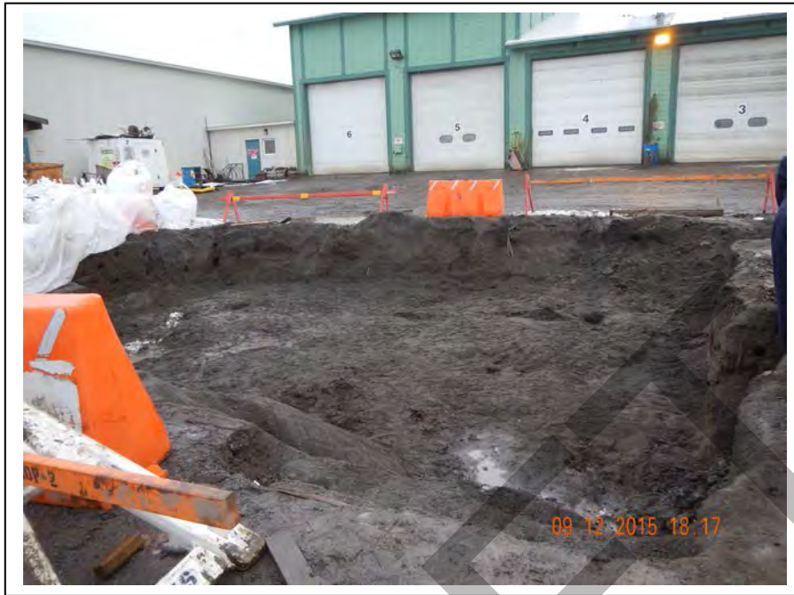
Photo 46: Excavation site at the conclusion of sampling; facing east (September 12, 2015).
