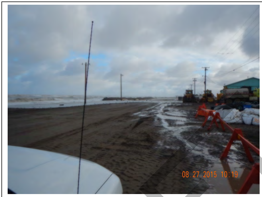
Photo 26: Ocean surf breaking over Stevenson Rd, adjacent to the excavation site (August 27, 2015).
