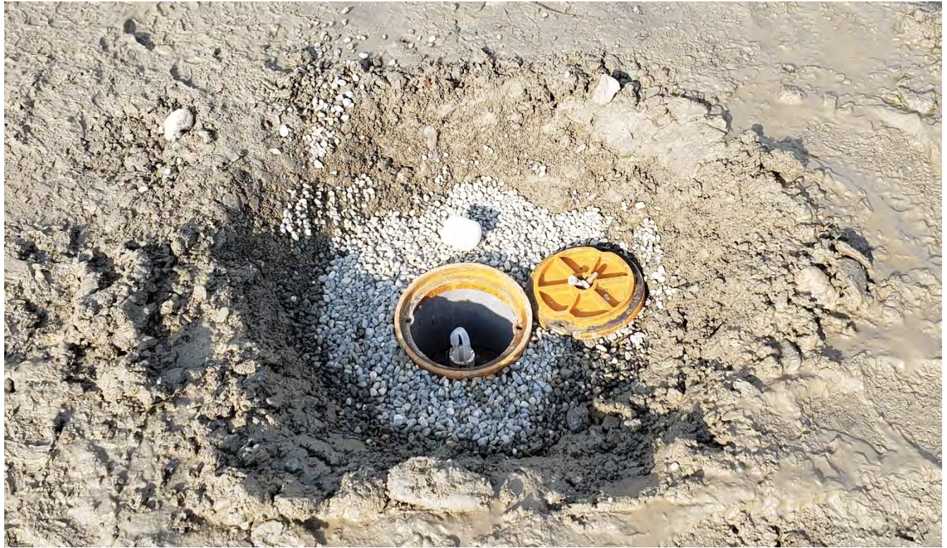
Photograph 5: Completed monitoring well MW-191 with buried flush-mount monument.
