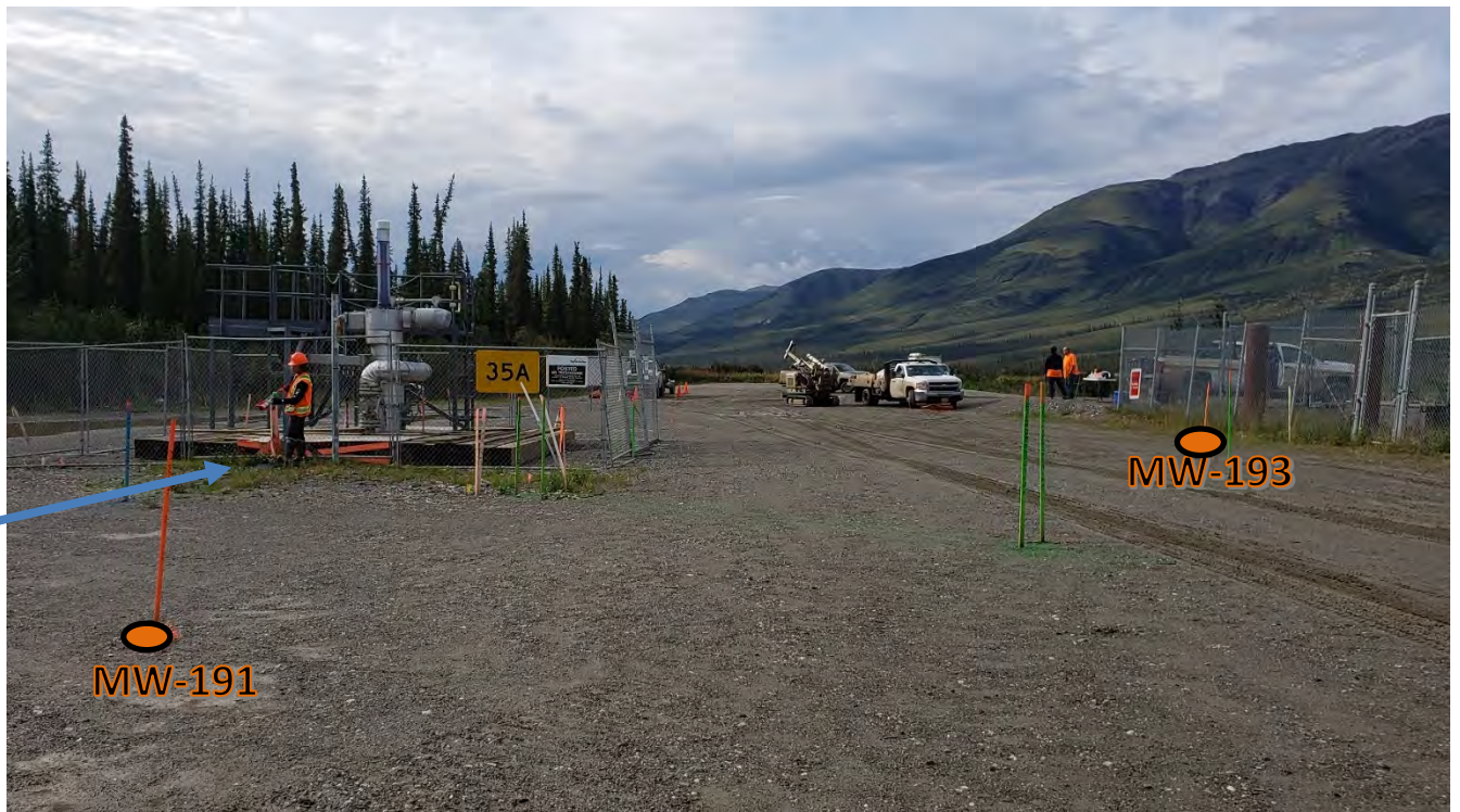
Photograph 2: MW-191 (left) and MW-193 (right) locations and pipeline flow direction (blue), view looking to pipeline south.
