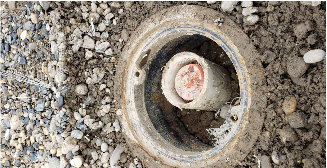
Monitoring Well MW-16R: The two-inch monitoring well casing (covered with an orange expandable cap) was cut down prior to sampling. Slits in the four inch well casing are visible above the gravel in the monument. (August 16, 2019).
