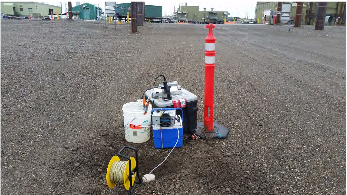
Photo 7: Monitoring Well MW-18: Well exposed in gravel pad, photograph facing south.
