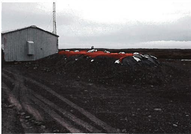
Photo 5. Completed biocell
