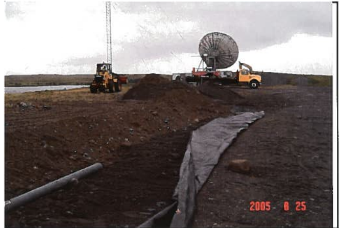
Photo 4. Biocell construction
