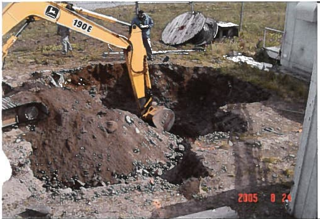
Photo 3. Soil excavation at E-TP-3 area
