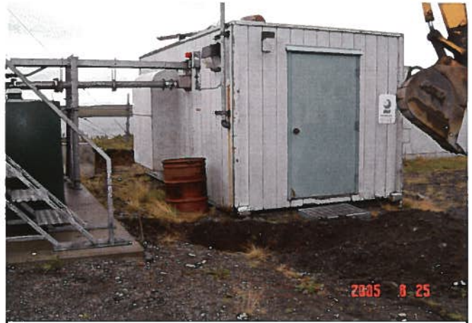
Photo 2. Excavation at E-TP-1 area.
