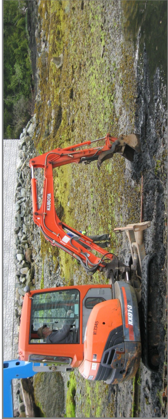
Removing contaminated sediment along the Marine Railways
