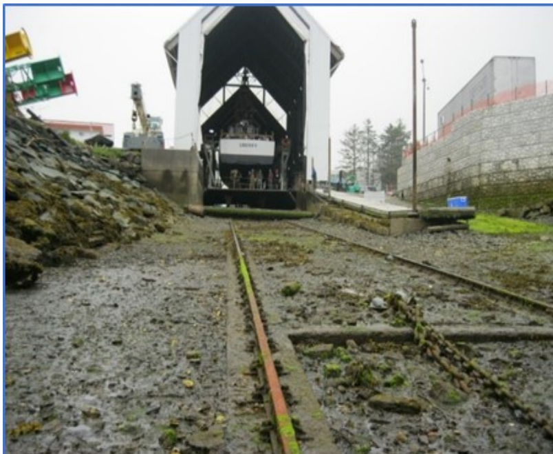
Inner Marine Ways sediment along the rails
