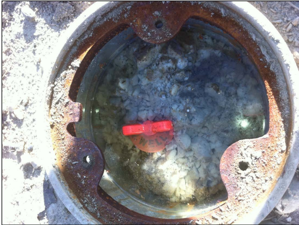
PHOTOGRAPH 5: VIEW OF WATER AND BENTONITE INSIDE THE MONUMENT OF MW-2 (SEPT 2011)
