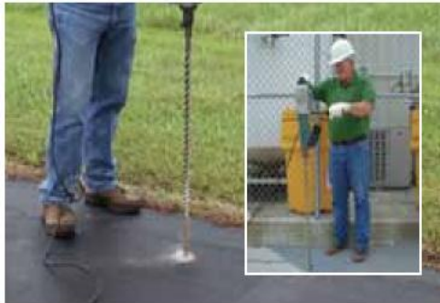
Hard surfaces - use a rotary hammer drill. Open ground - use rotary hammer drill, slam bar & tile probe, or hammer and steel rod
