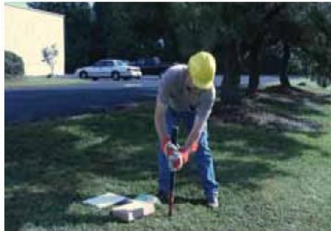
Make 0.5 to 1 inch hole 36 inches (1m) deep
