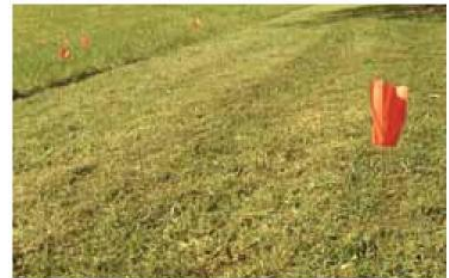
Lay out sampling grid prior to drilling holes
