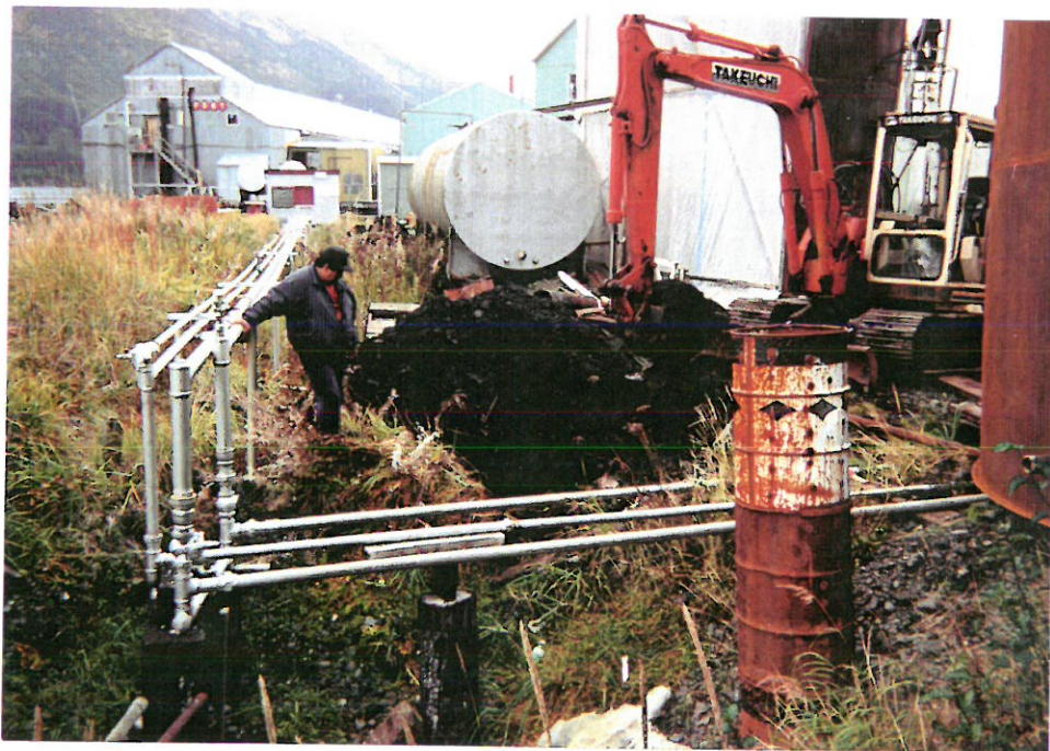
Test pit number five, adjacent to excavation "C"
