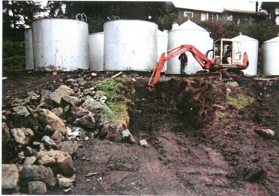
Test pit number six, adjacent to embankment
