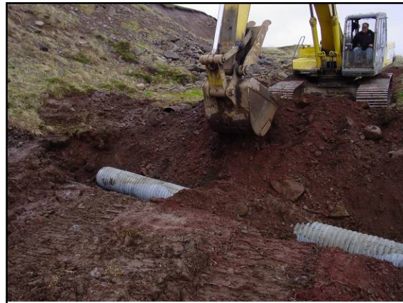
Photo 4. The second washout was widened and a culvert installed.
