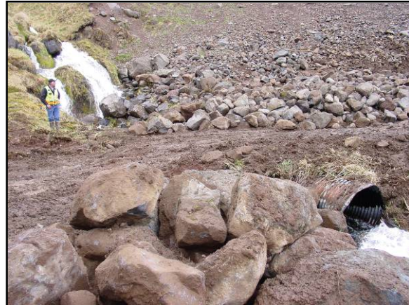
Photo 3. The culvert underlying the landslide was exposed on the uphill side.
