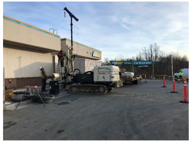
Photo 2: "Drilling RW 19-1 Well with Geoprobe 8040DT track mounted drilling rig operated by GeoTek Alaska
