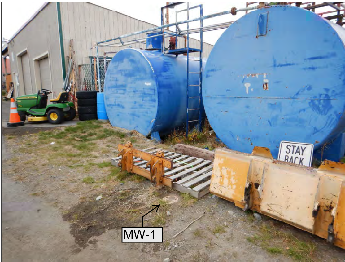
Photo: 3 Time: 1839 Date: 9/6/2019 Direction: Northwest Subject: MW-1, west and east ASTs.
