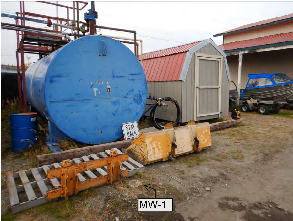
Photo: 2 Time: 1839 Date: 9/17/2019 Direction: East Subject: MW-1, east AST.
