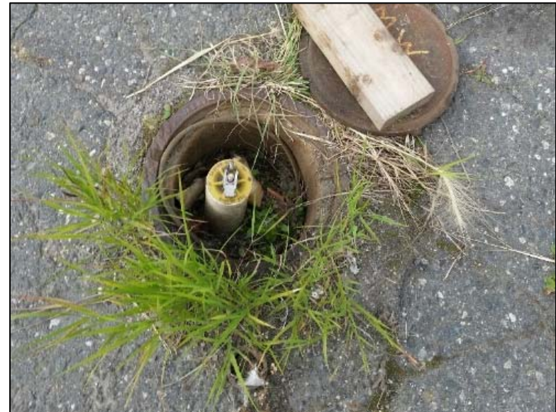
MWB09 inner PVC casing found in good condition.
