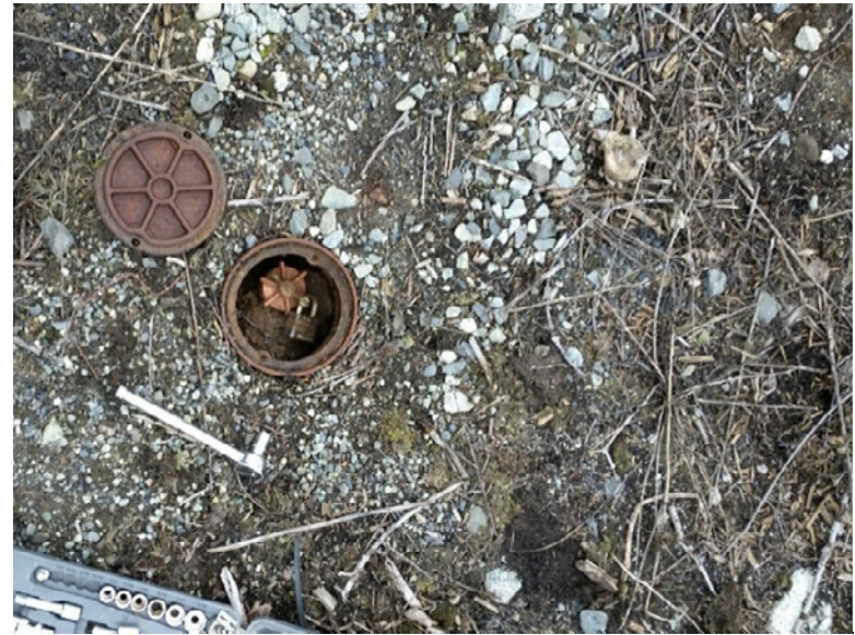
Locked well cap of MWE05.
