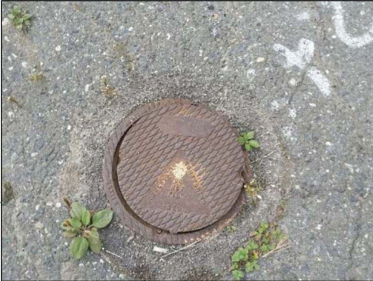
MW24 outer protective casing cap.
