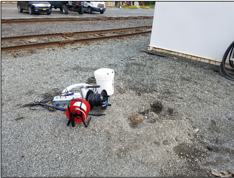
Flush mount monitoring well MWE04; looking northeast.
