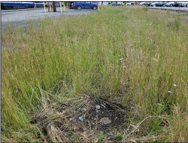
Flush mount monitoring well MWE20; looking east.
