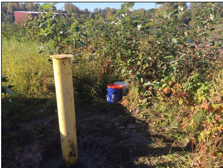
Monitoring well MWE11 and stored purge water; looking southwest.
