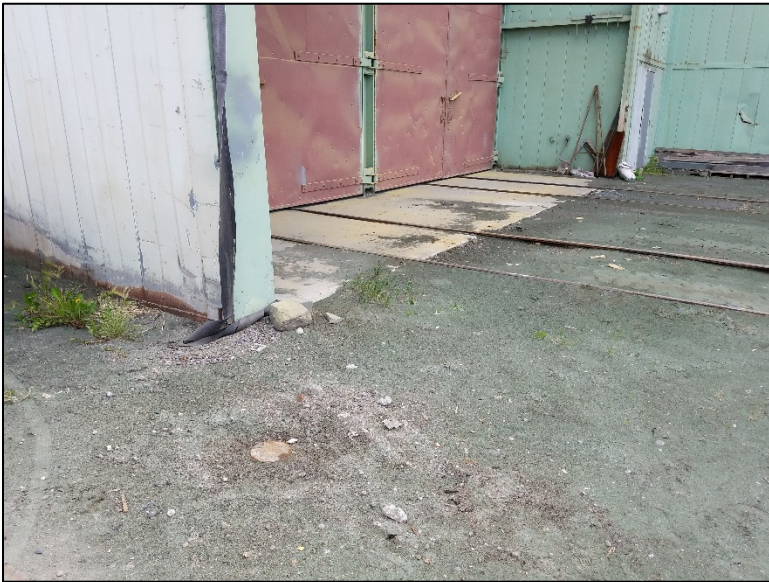
Flush mount monitoring well MWC01; looking southeast.
