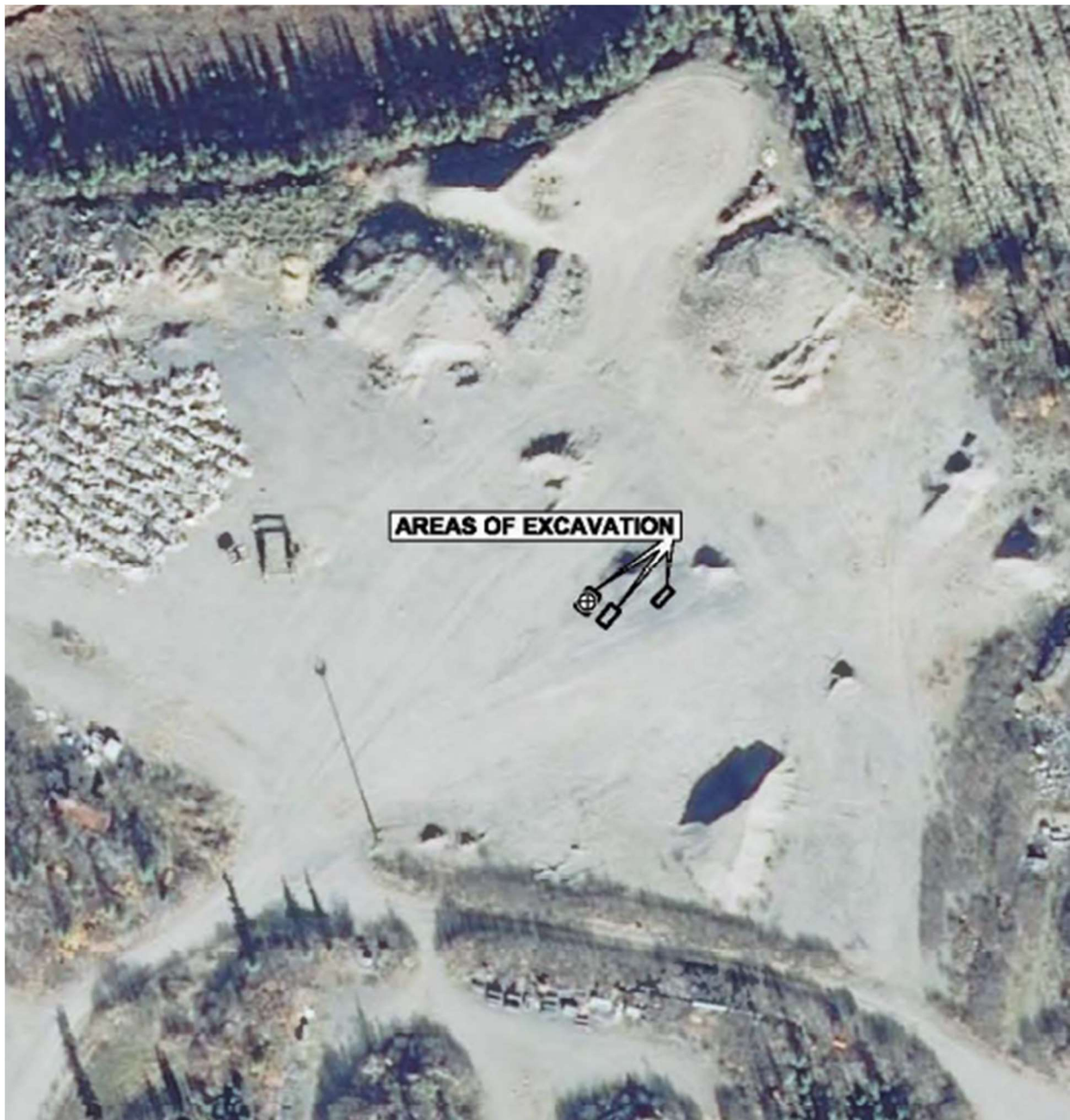
Figure 2: Aerial detail of DA034 where excavations occurred in 2014.
