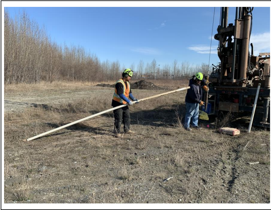
Photo 3: Looking north, the Well MW30 casing removed from the ground. (May 5, 2020)
