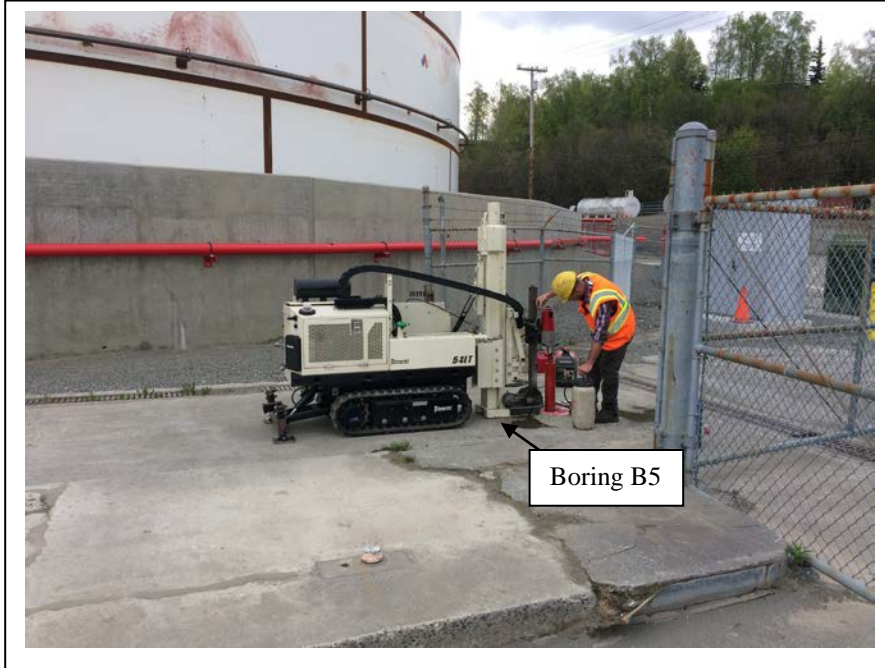
Photo 5: Concrete coring at Boring B5; looking southeast. (May 17, 2017)
