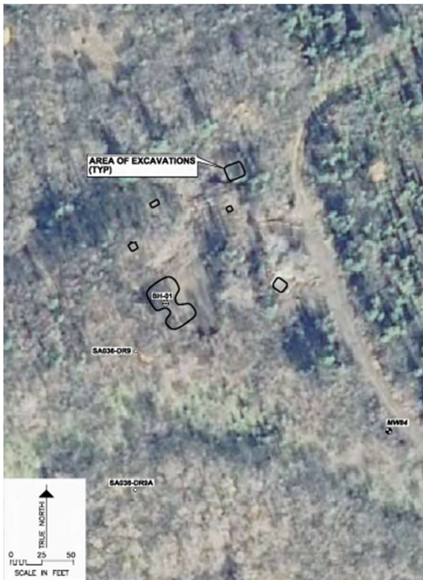
Figure 4: 2012 photograph detailing excavations at SA036-DR9.
