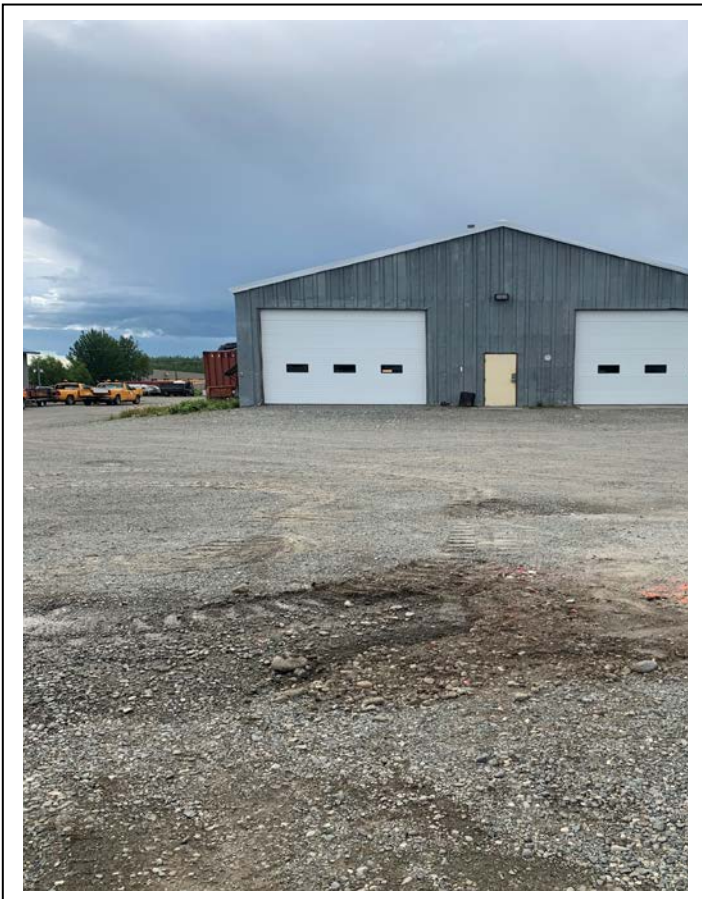
Photo 4: Looking west at the location of Boring B2. (June 7, 2019)
