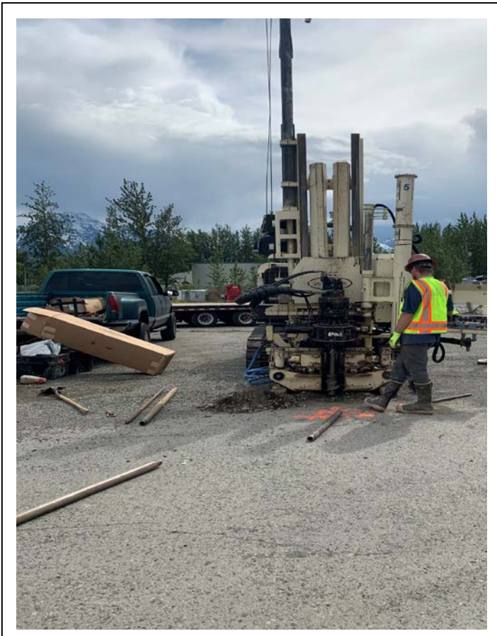
Photo 3: Looking south at the advancement of Boring B2. (June 7, 2019)
