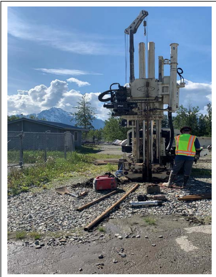
Photo 1: Looking south at the advancement of Boring B1. (June 7, 2019)
