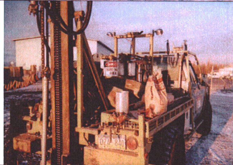
Photo 5: Removal of well MW-5.
