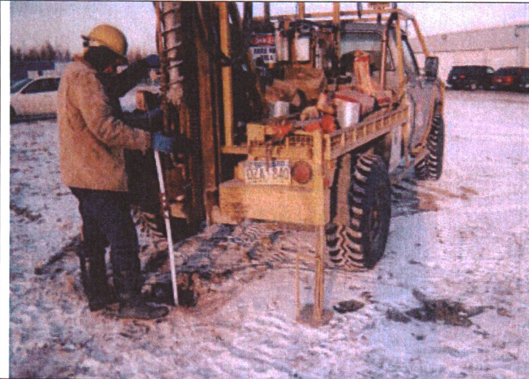
Photo 4: Removal of Well MW-1.
