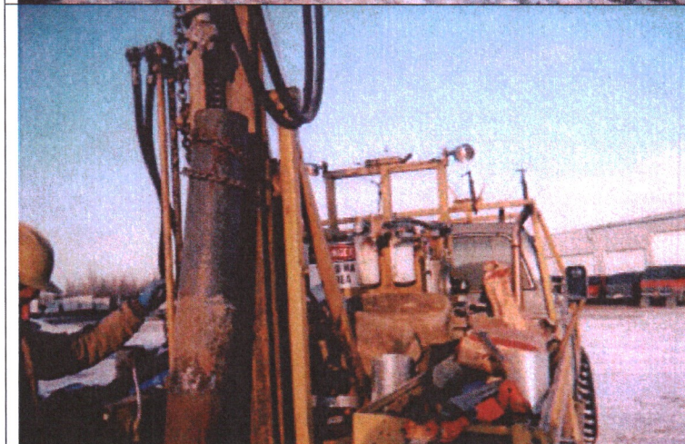
Photo 3: Removal of well MW-1 monument.
