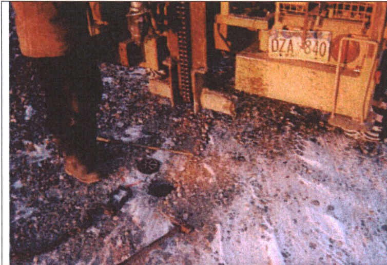
Photo 1: Well MW-5 prior to it's removal.
