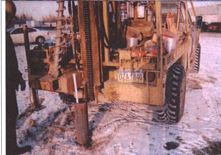
Photo 2: Well MW-1 Prior to its removal.
