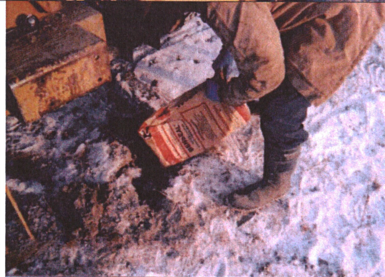
Photo 6: Applying Benseal Bentonite grout after removal of well MW-1.
