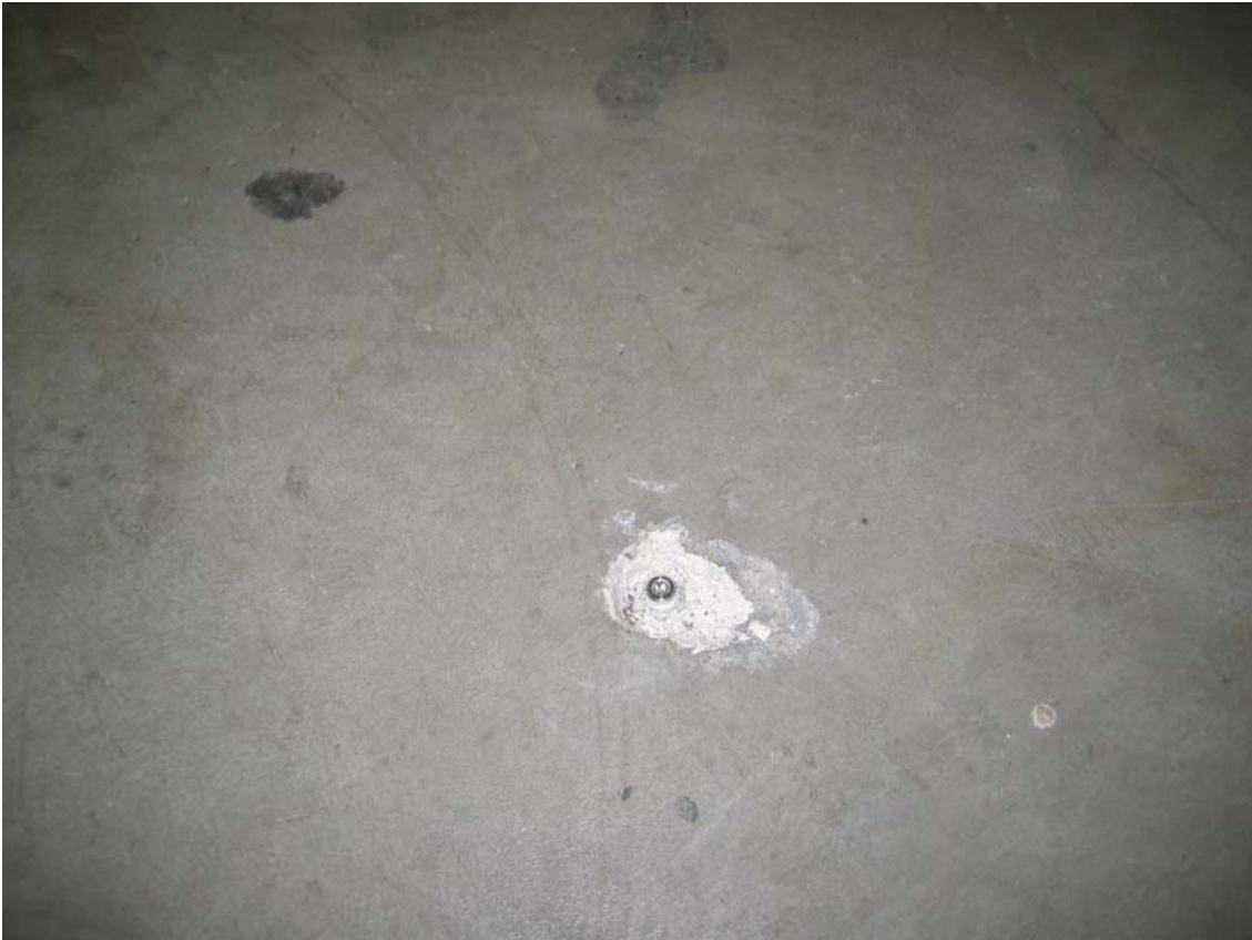
Photograph 3 A sub-slab sampling point cemented into the floor at LP-072.
