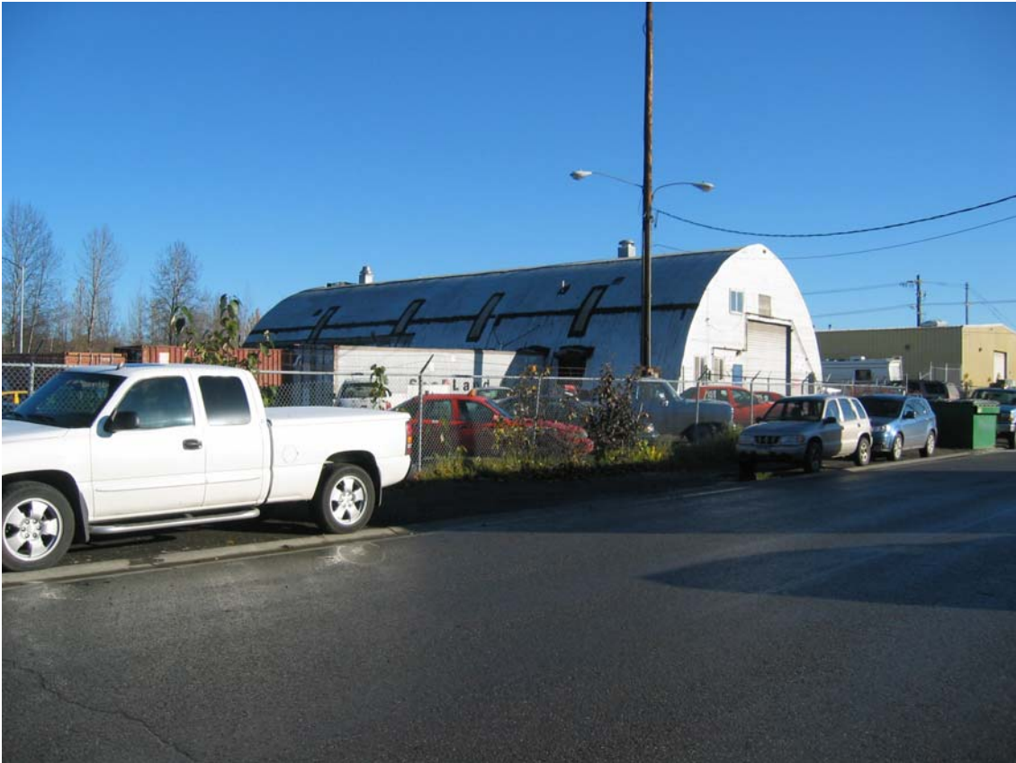
Photograph 5 LP-125 from the southwest looking toward the northeast.
