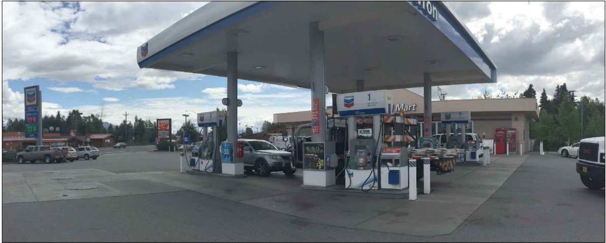
1. Site overview, looking southeast
