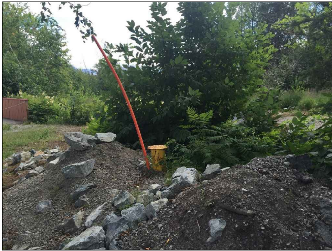
2. Offsite well MW-8
