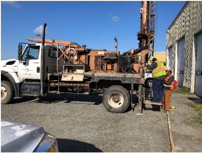
Photo 1. A truck mounted drill rig was used to decommission the well
