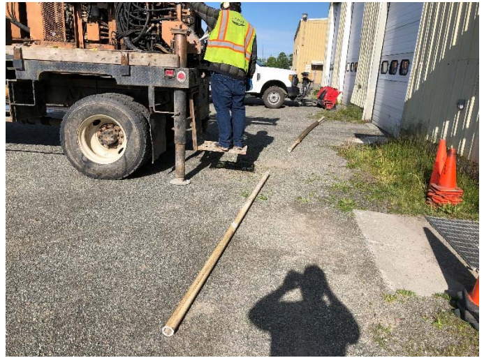
Photo 2. The full casing of the well was removed
