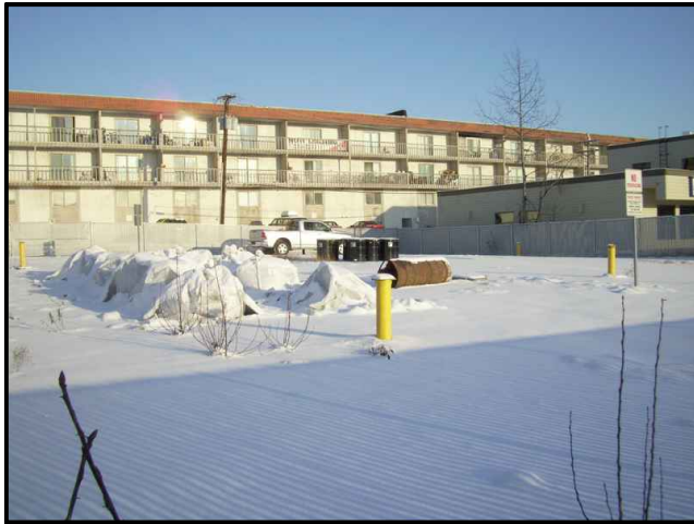
1. Site layout looking Northeast
