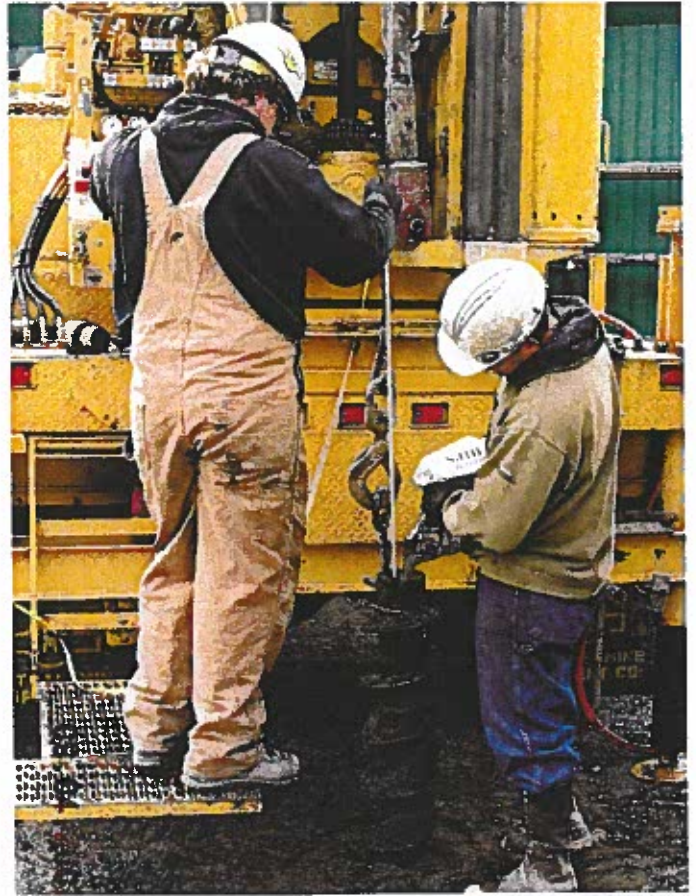
Constructing air sparge well
