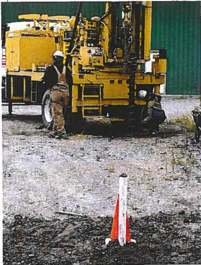
Drilling hole for air sparge well
