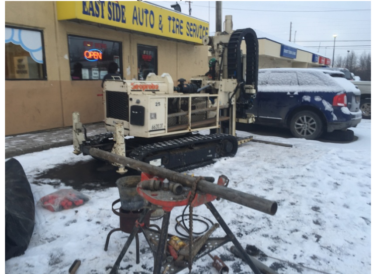
Photo 4. Soil Boring SB6B (looking Northwest)
