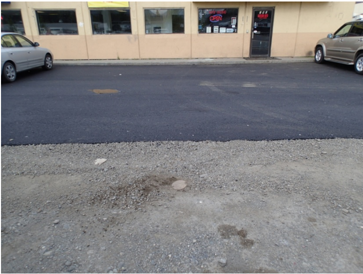
Photo 1. MW7 (looking West)
