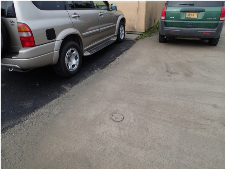
Photo 3. MW26 (looking West)
