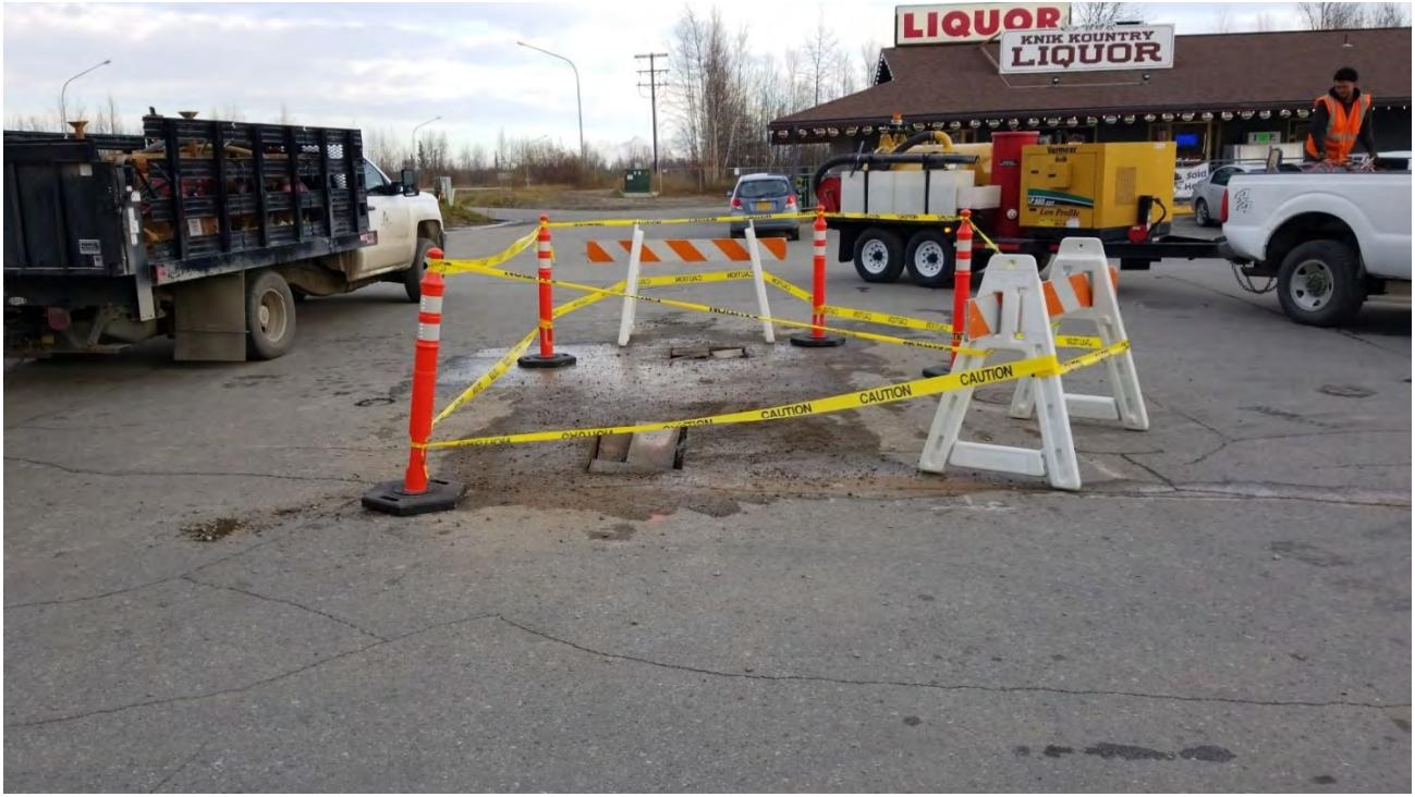
RW20-1 and RW20-2 locations with cut asphalt prior to drilling and barricaded.
