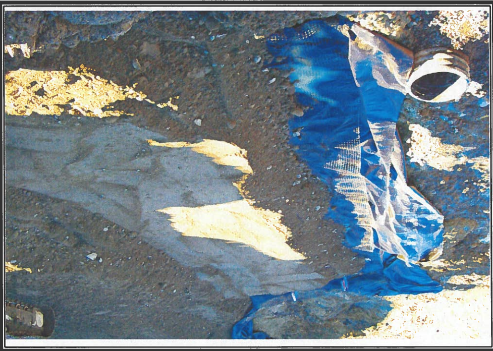
Photo 17: Compaction near the north wall of the excavation.
