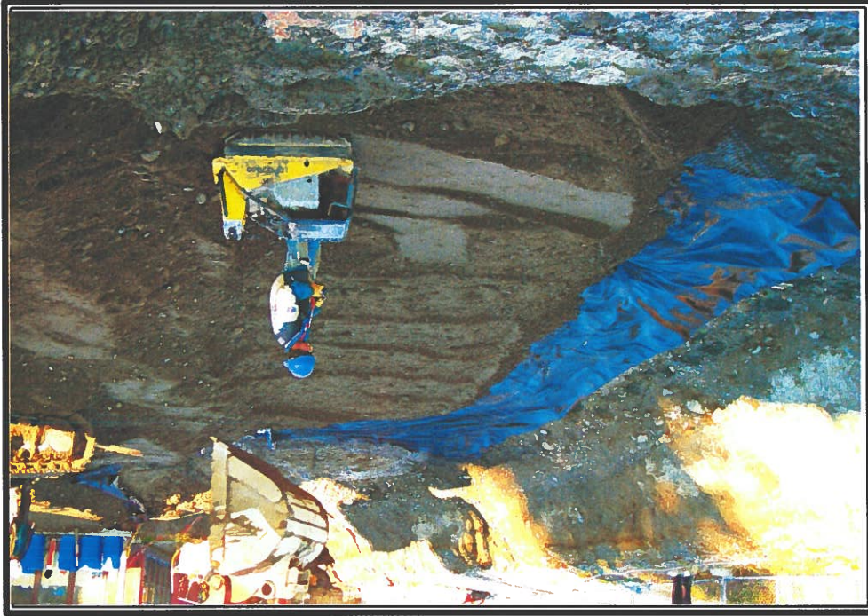
Photo 13: Placement of filter fabric along the south end of the excavation.
