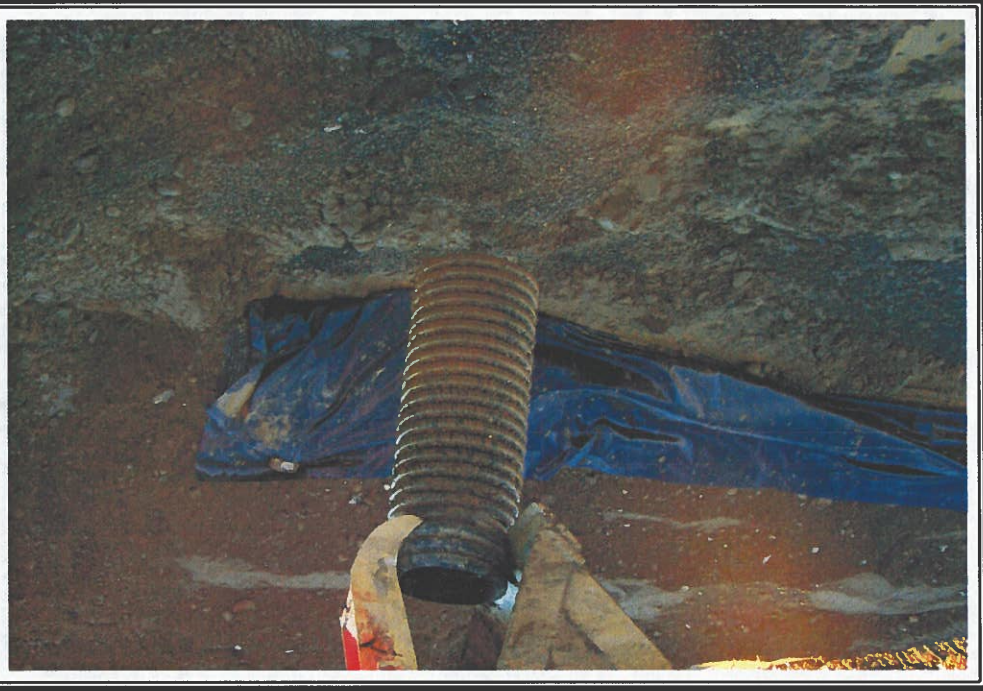
Photo 18: Removal of sump pipe initially used to stabilize the excavation.
