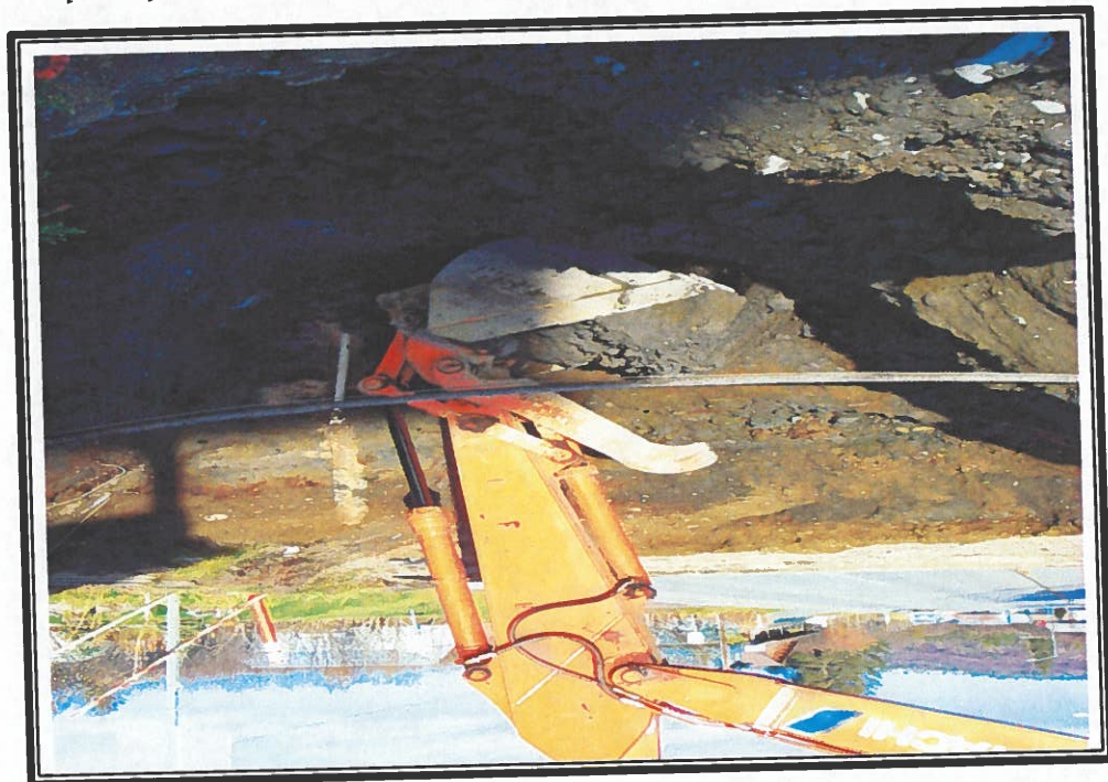
Photo 7: Excavation activities around an existing electrical line, along the north side of the excavation.
