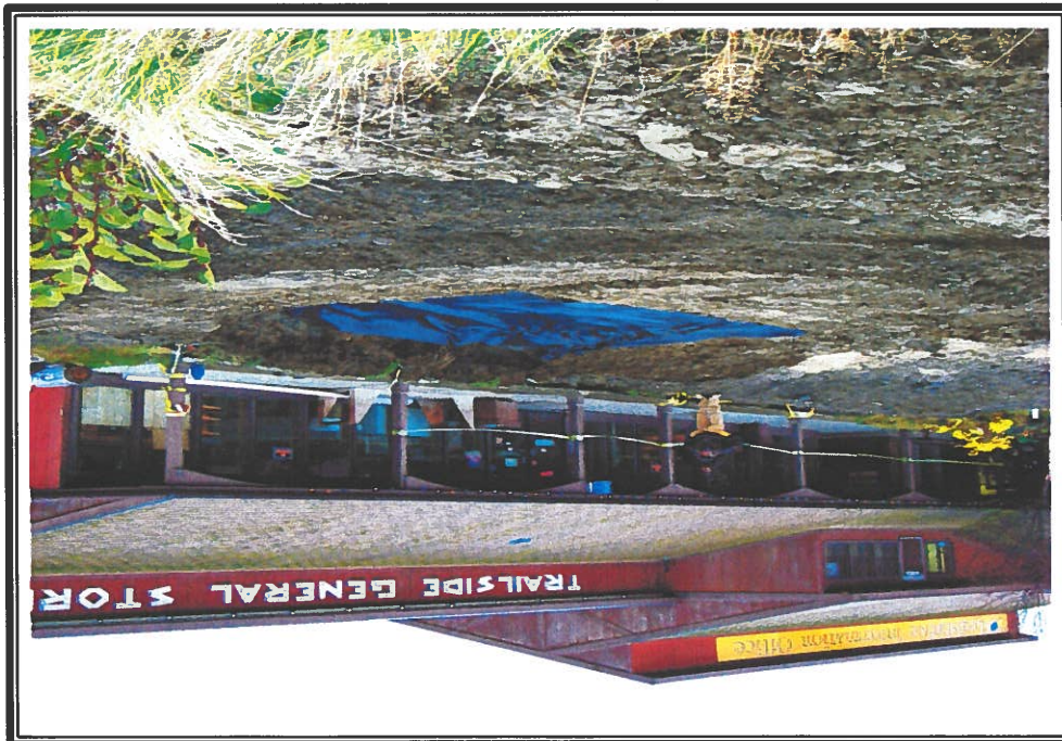
Photo 13: Placement of filter fabric along the south end of the excavation.
