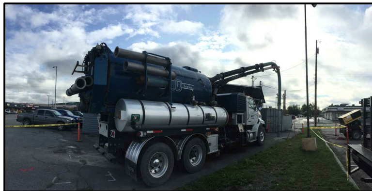
PHOTO 4: VACUUM TRUCK AT SB17-1 FACING SOUTHEAST
