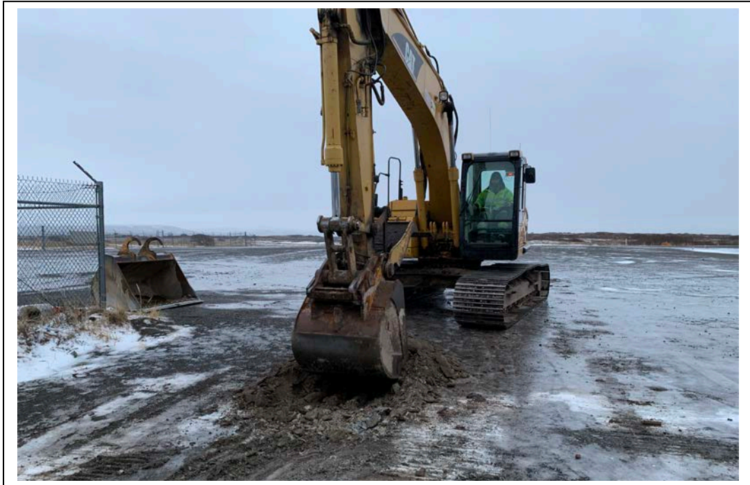
Photo 1: Looking south at the advancement of Test Pit TP1. (November 5, 2020)
