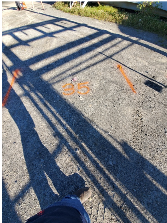
Photo 2: Boiler Building Trench Excavation – Section -35 along the trench transect.
