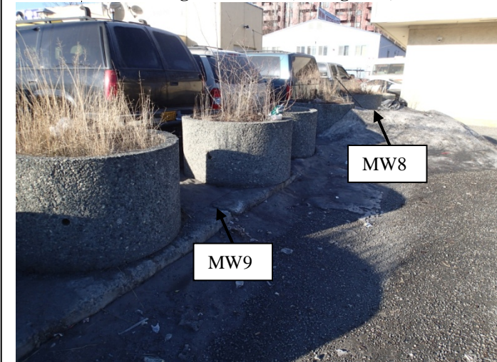
Photo 3. Monitoring Well MW8 and MW9 (Facing SW)
