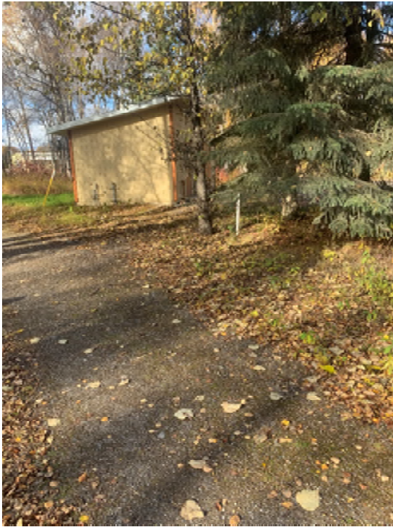
FG-14 surrounding Facing North
