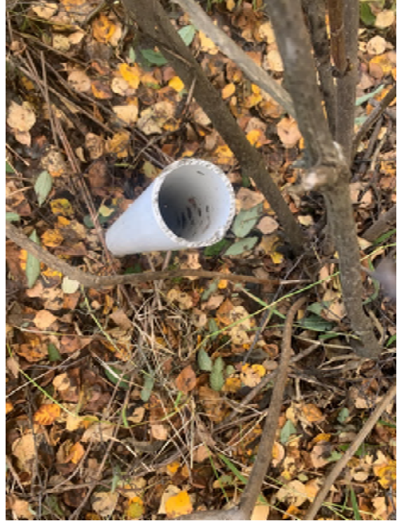
Closeup/overhead of HOS-5
