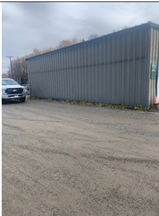
Assumed former location of HOS-3 Facing East
