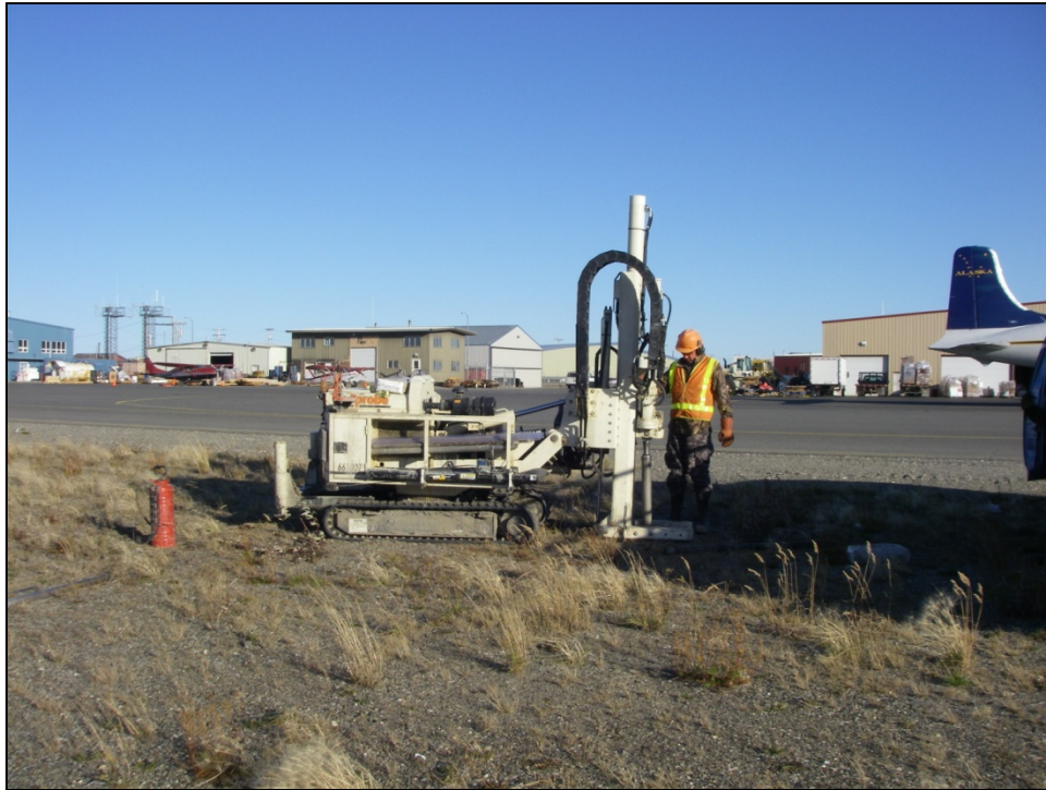
PHOTOGRAPH 1: KOTZEBUE UST SITE, VIEW NORTH. DRILLING MW-1R WELL. 23 SEPTEMBER 2010. 10:48
