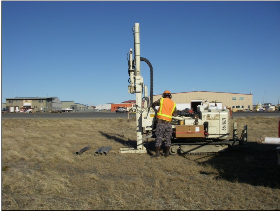
PHOTOGRAPH 3: KOTZEBUE UST SITE, VIEW NORTH. DRILLING MW-3R. 23 SEPTEMBER 2010.
