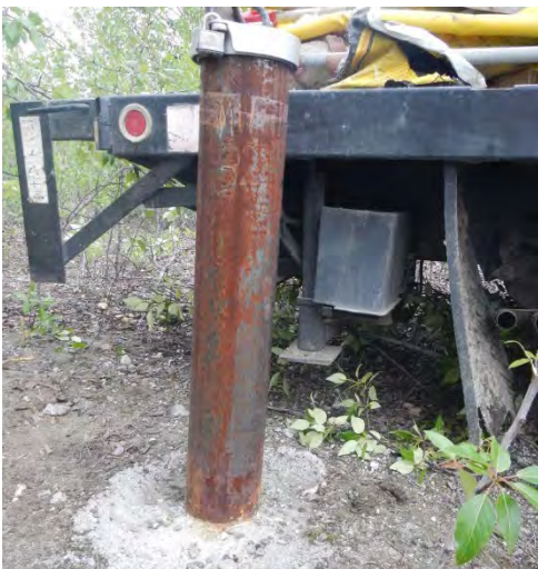
MW-32 after repair.
