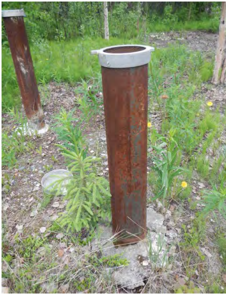
MW-27 before repair.
