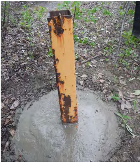
MW-4 after repair.
