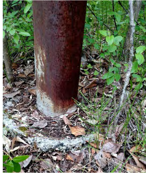
Frost-jacking at MW-18.
