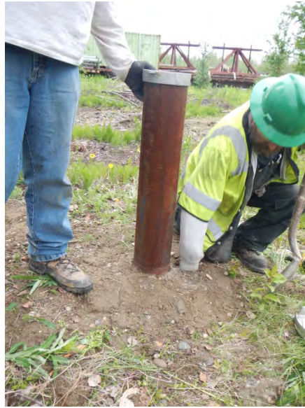
MW-27 after repair.
