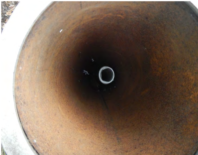
Inside MW-29 after removing portion of bent casing.
