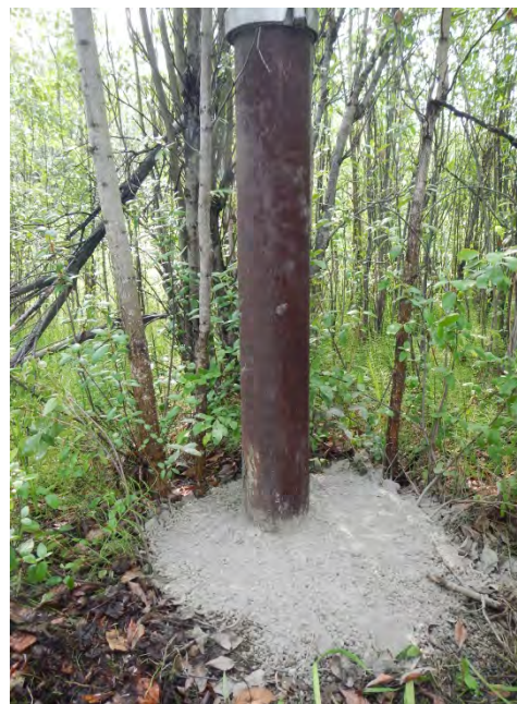
MW-18 after repair.
