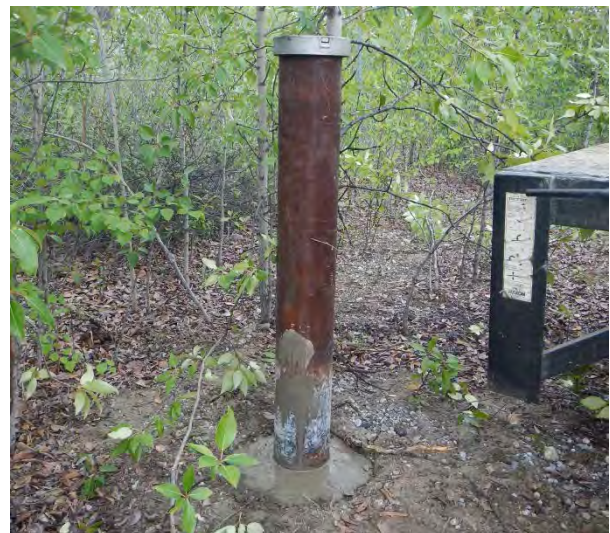
MW-31 after repair.
