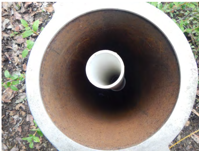
Inside MW-29 after repair.
