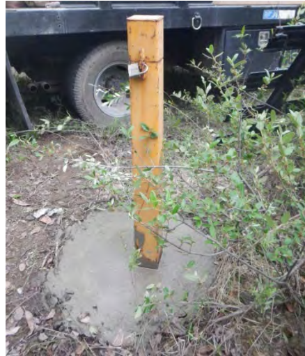
MW-5 after repair.
