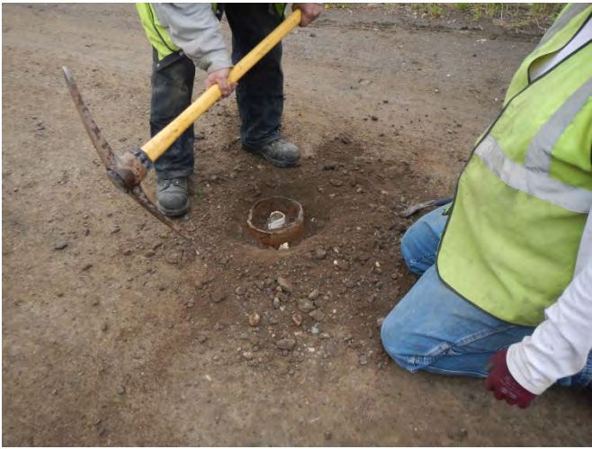
Digging out remaining portions of MW-12.
