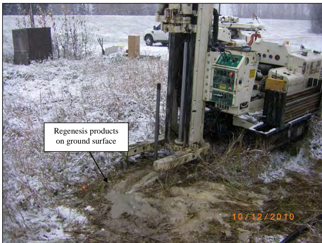
Completed injection point prior to removing injection rods (view to the northwest)
