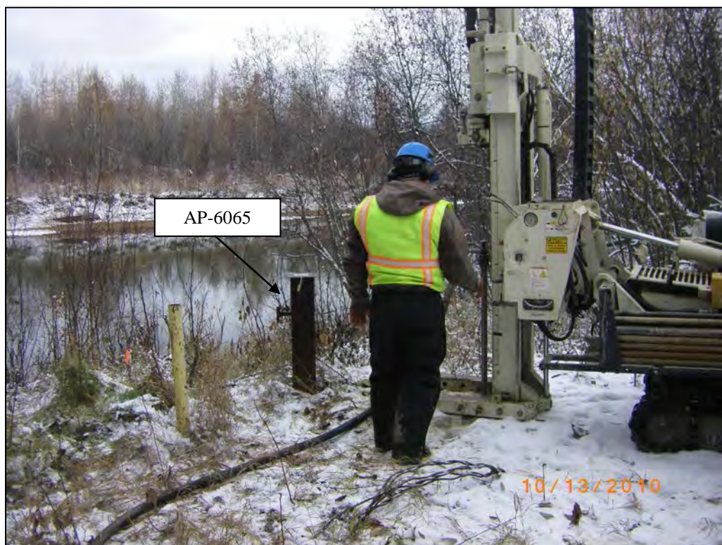
Completing an injection point near AP-6065 (view to the southeast)
