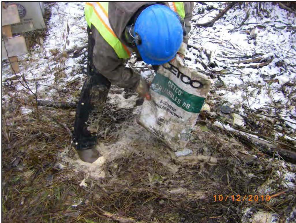
Filling a completed injection point with bentonite crumbles (view N/A)
